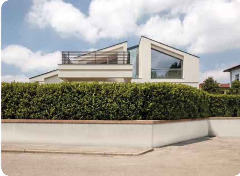
PROGETTO | PROJECT HPBA | Houseporch Albinea (RE) PROGETTISTI | DESIGN TEAM Natoffice Arch. Christian Gasparini
