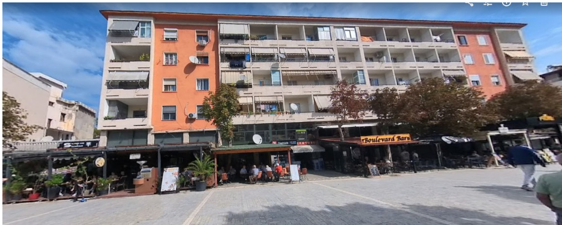
Post-war apartment blocks as part of the projected extension in the buffer zone
