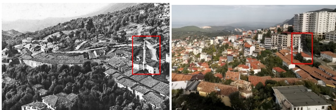
Figure 5-10 (left) view of the bazaar after WWII highlighting the bazaar mosque as common element in both pictures, source: Technical Archive of the National Institute for Cultural Heritage, (right) view of the Bazaar in 2007, source: author
