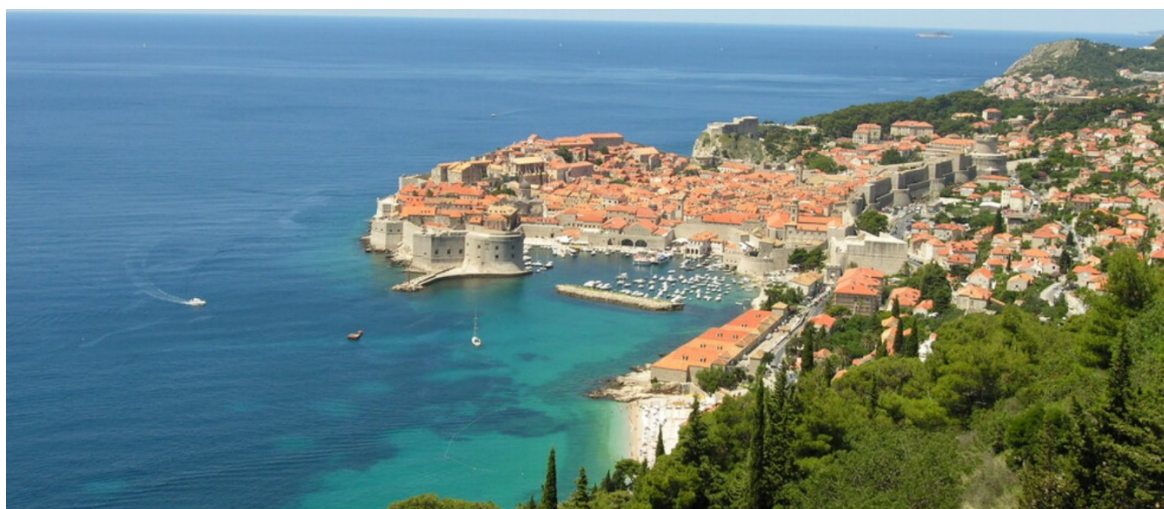
Figure 5-54 – View of the Old city of Dubrovnik. Source: Unesco, authored by Bandarin F. (2005) 109
