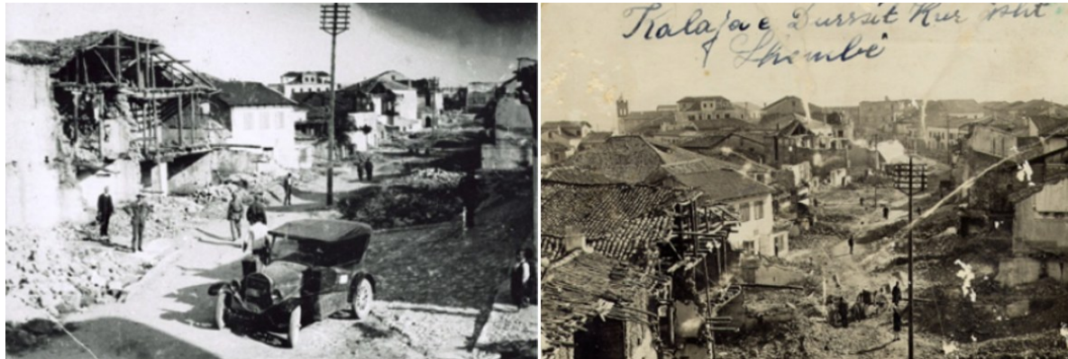
Figure 5-30 - Images showing the destructions of the 1926 earthquake in the neighbourhood within the fortification walls, Durrës 99
