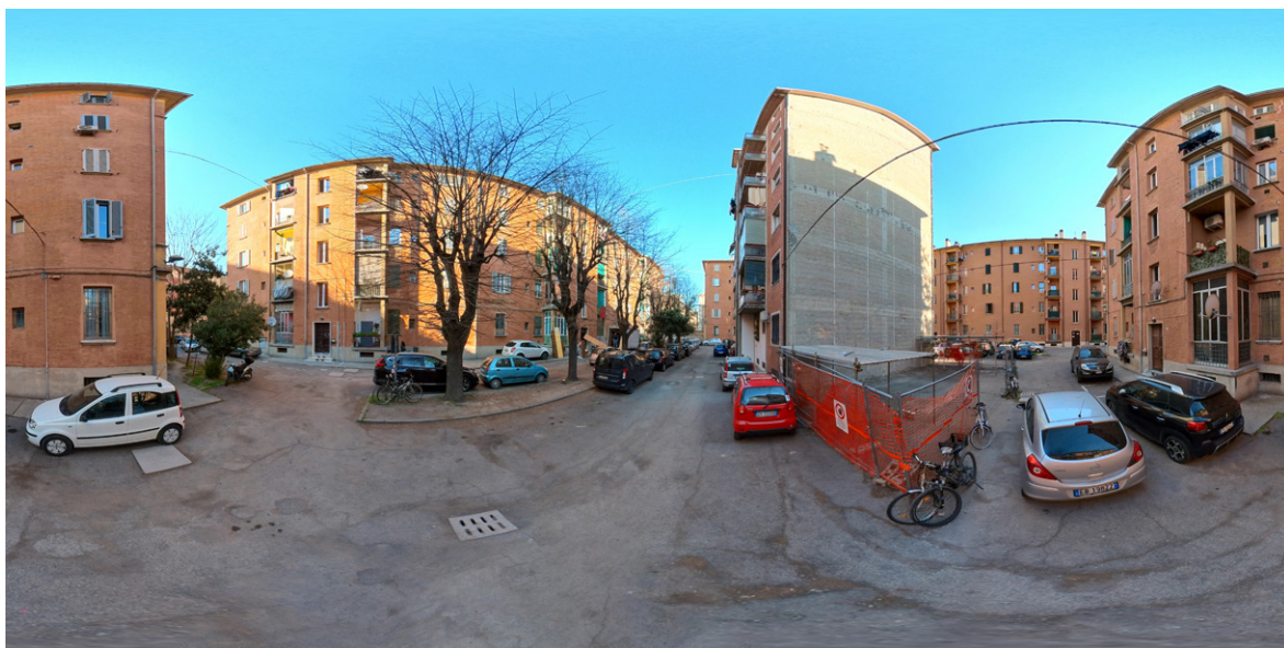
Fig 22- Using 360° images was crucial to reducing the number of case study inspections (conducted during the first wave of Covid 19). The photos are used for documentation purposes to check the positioning of elements in the model visually.
