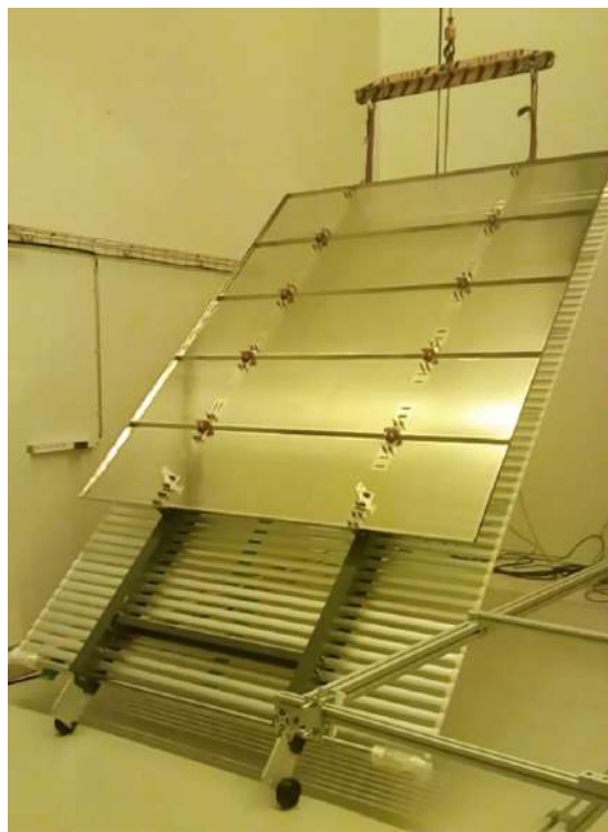
Figure 18. Lifting of a Top FC module for subsequent installation on the CPA panel. The side of the FC module that is lifted will attach to the CPA while the other side (bottom side) is connected with latches to the APA.
