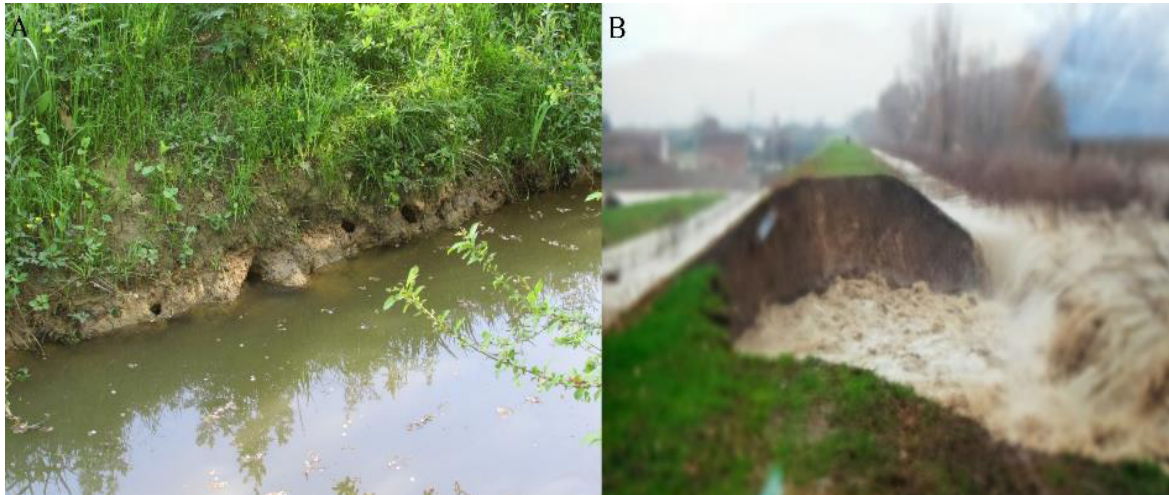
Figure 1: A = Typical burrows produced by Procambarus clarkii on irrigation ditches; B = Due to the burrowing activity of Procambarus clarkii broken levee alongside the river Secchia (Emilia Romana, Italy).
