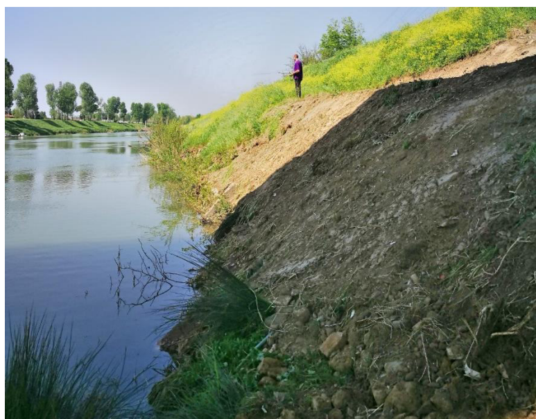
Figure 1: North riverbank of the Arno river after mechanical removal of vegetation.
