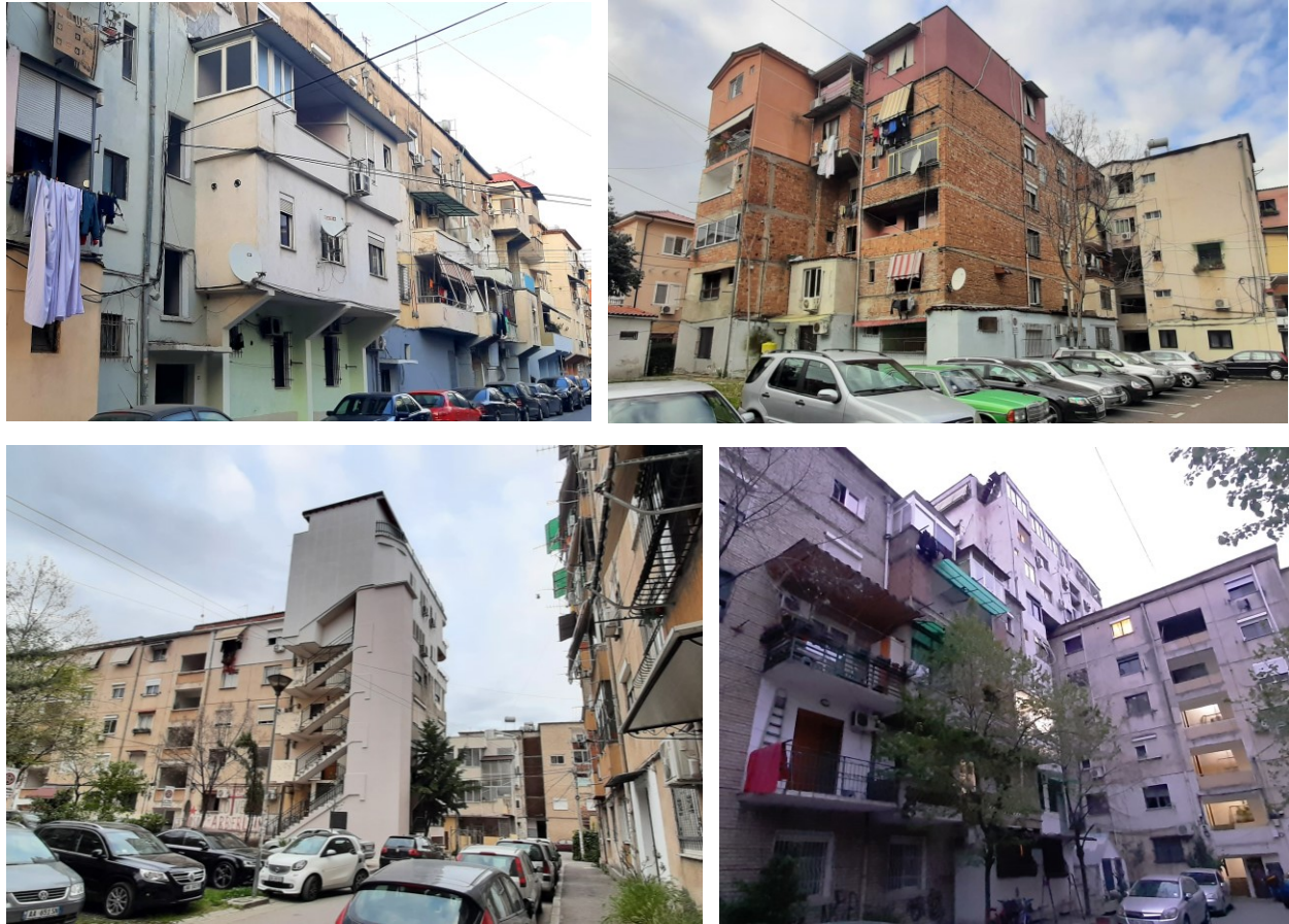
Figure 59. Volumetric transformations, "parasite volumes" type, in residential buildings of the '70s-'80s in Tirana.
