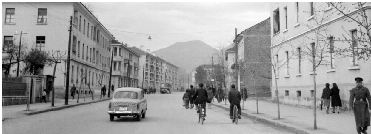
Figura 31. New constructions on "Bajram Curri" street.
