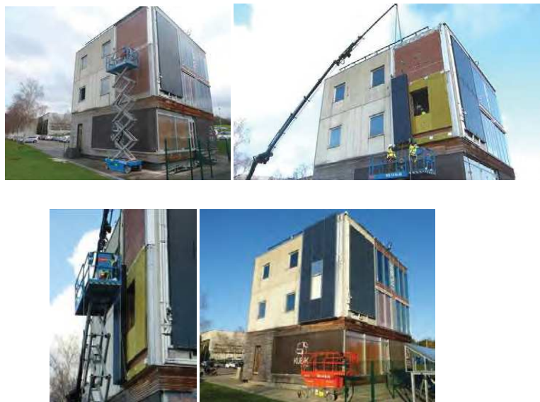
Figure 5: Installation of the RenoZEB Plug and Play façade system
