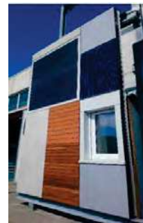
Figure 3: RenoZEB envelope system's wall composition (left) and Mock-up of the RenoZEB facade module (right)
