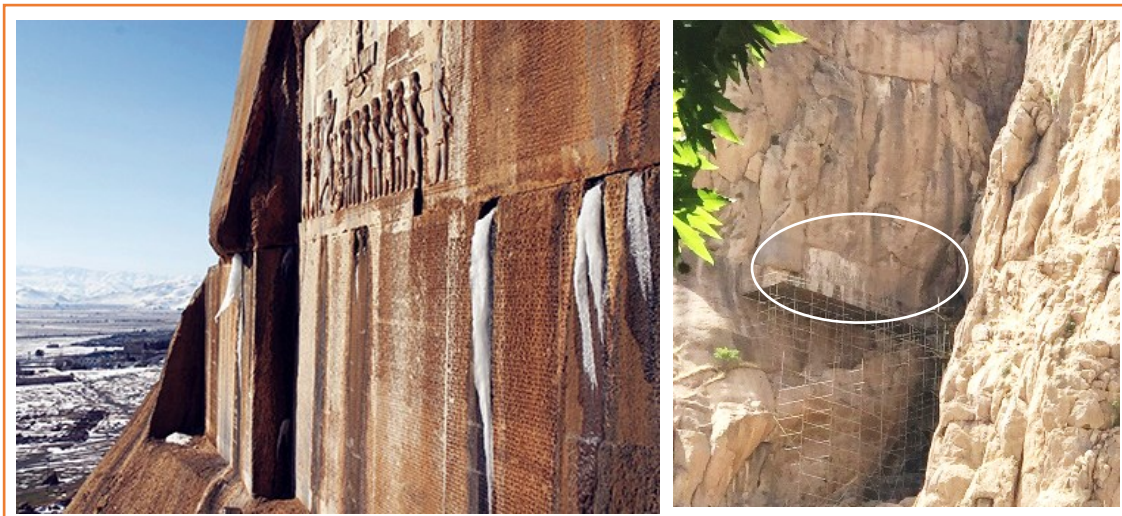
Figure 13:Underground water flow in D.I.B- https://www.koochar.com/en/wiki/iran/cities-of-iran/kermanshah-
