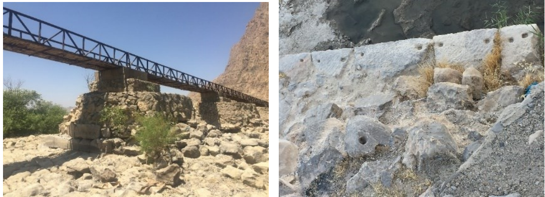
Figure 23:Khosrow Bridges bed level and piers, Source: Author,2018
