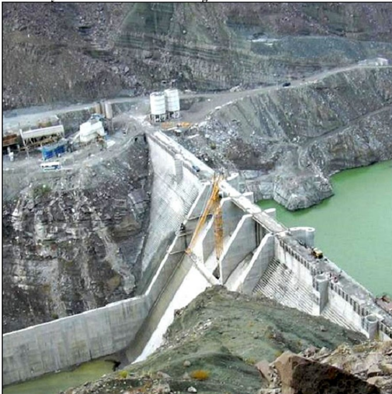
4: Garin Dam on Gamasyab in Nahavand, Hamadan
