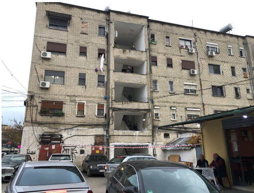
Figure 3-11 Photo of the building 77/11
