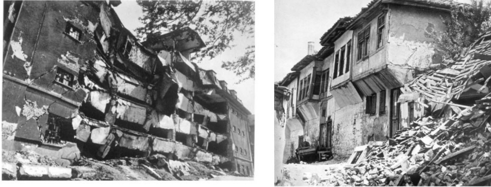
Figure 2-3 Images of damaged buildings from 1963 Shkupi earthquake (Source: Petrovski, 2004)
