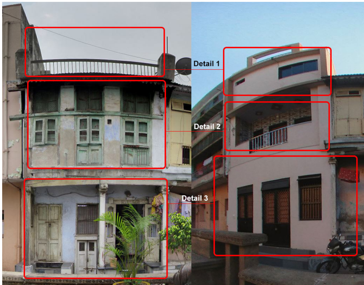
Figure 29: Detail of the two facades and main changes. The building has a sharing wall system: this means that on the other three sides it can not grow.
