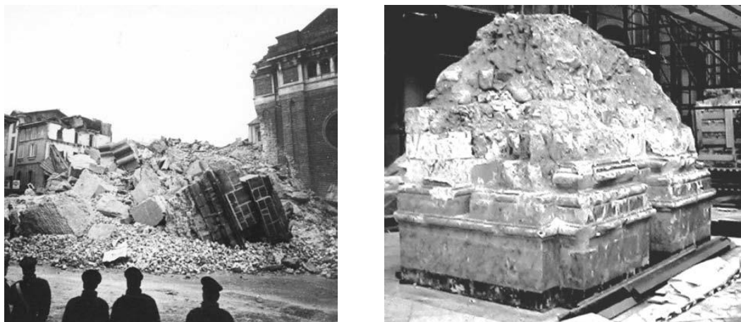
Figure 5.1: some examples of the collapse of heritage masonry building: a) the ruin of Civic Tower of Pavia in 1989 after the collapse (image from Binda, Anzani, and Saisi (2008)), b) a damaged pillar of the Noto Cathedral (image from Saisi et al. (2008)).
