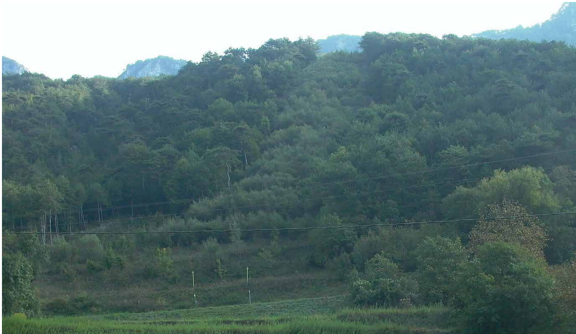
Figure 2.61: The trail of the SNAM's pipeline still visible five years after the works completion. (Source: ILCEV, www.ilcev.it )
