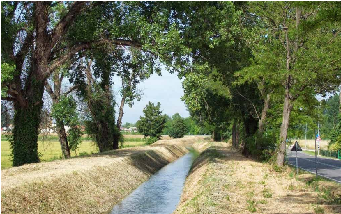
Figure 4.2: The 'Mills' Canal' managed by the CBRO Consortium and declared by the Emilia-Romagna Region, ecologic corridor in contrast with maintenance operations which require, as in the picture, enough space on the banks to be performed.
