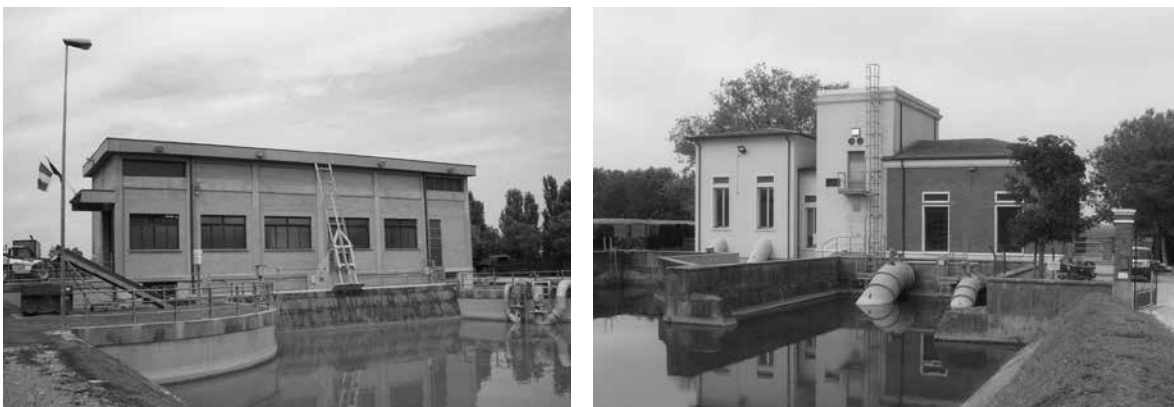
Figure 3.35: Below, images of two dewatering stations managed by the Consortium; on the right, the '1° Bacino Mandriole', on the left, the 'Tratturo'. (Source: CBRO Documentation Archive)
