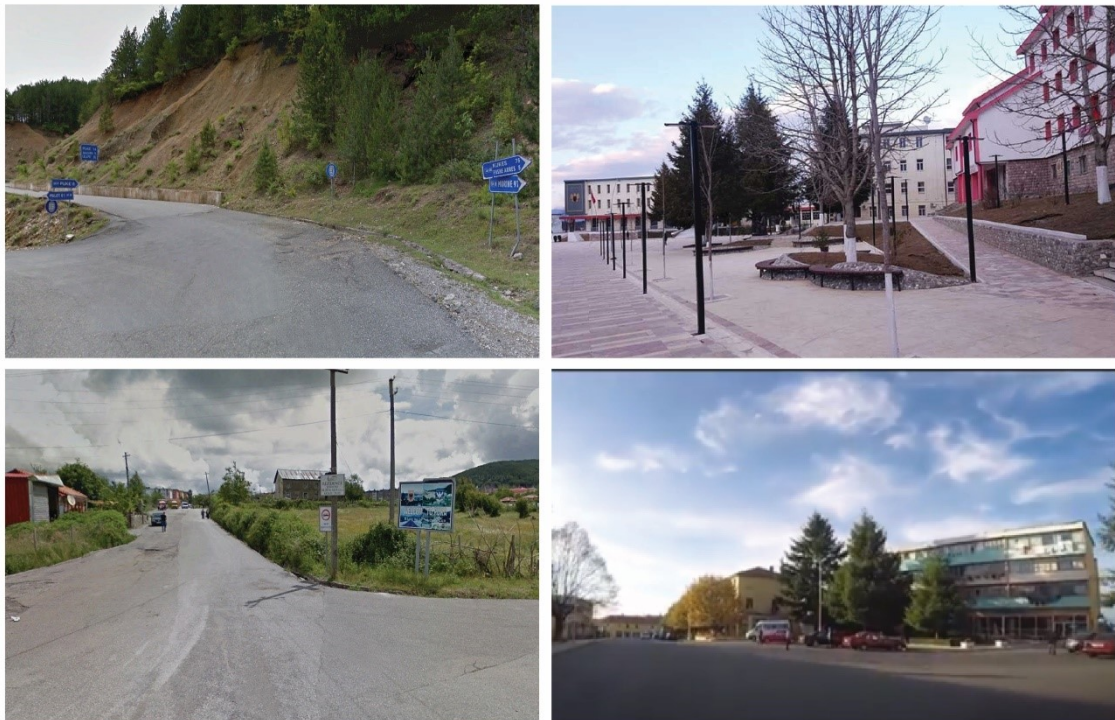
Figure 62. The Pukë settlements visual condition. (Source: the author).
