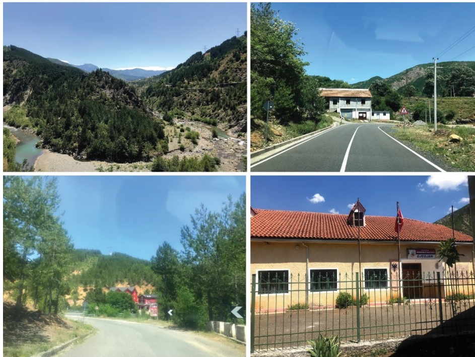
Figure 55. The Gjegjan settlements visual condition. (Source: the author)
