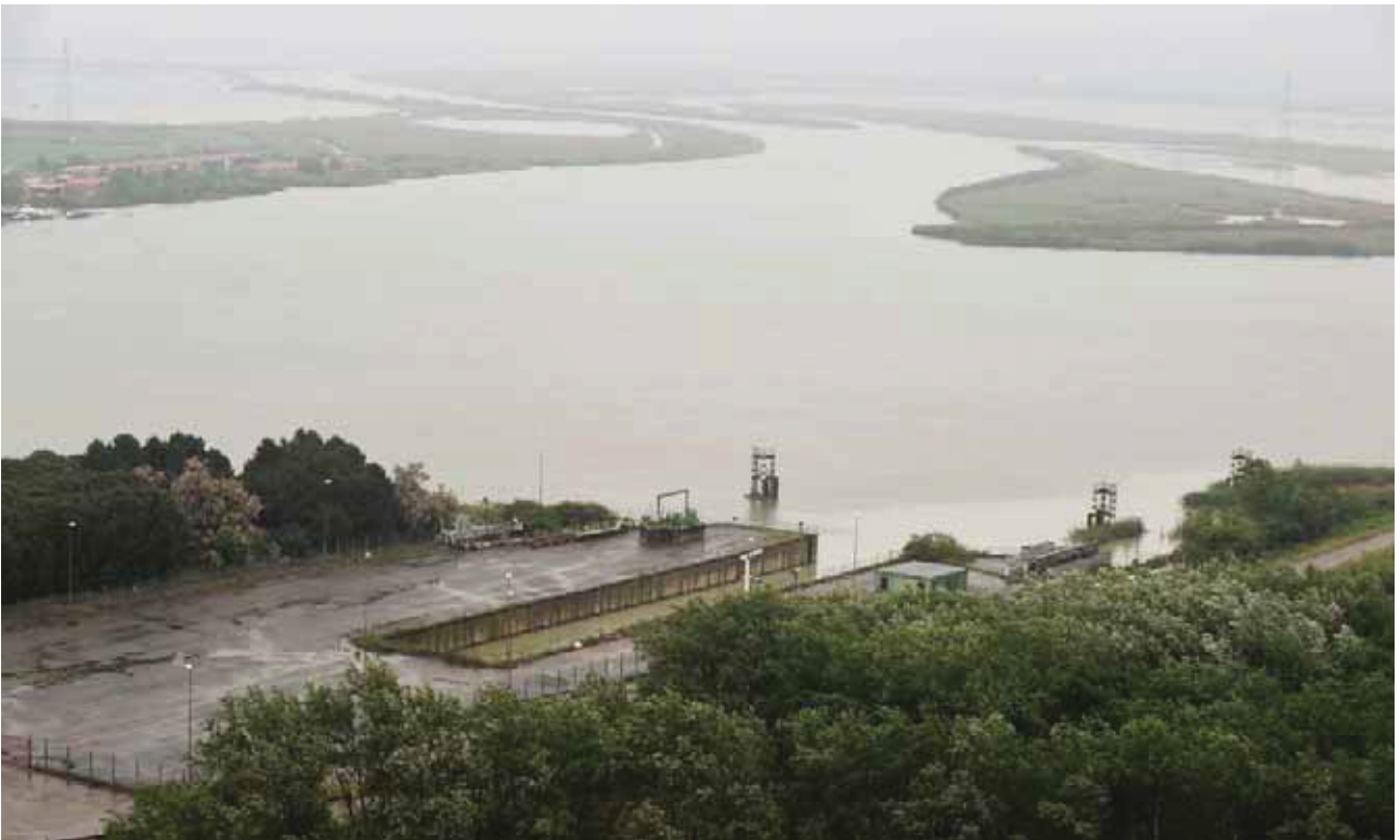
Fig. 228 The quayside for oil barges (source: Enel)
