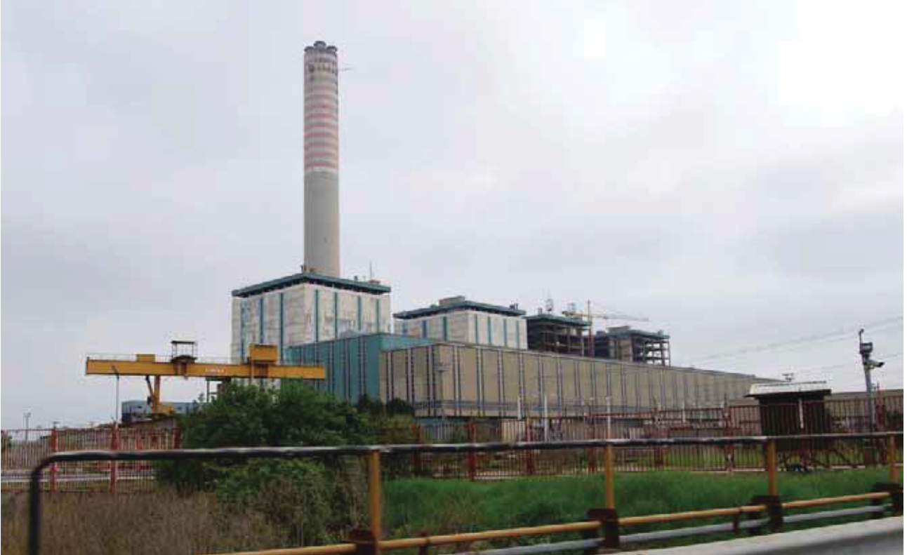
Fig. 227 Polesine Camerini thermal power plant (source: Enel)
