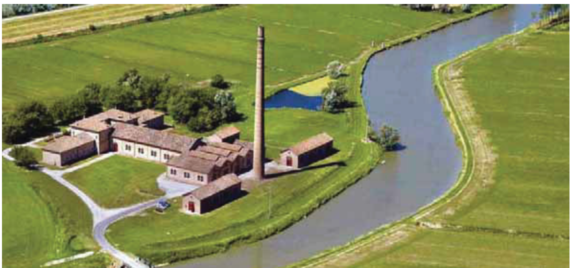
Fig. 202 Ca' Vendramin water pumping station (source: Quaderni Ca' Vendramin n.0)
