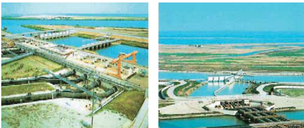
Fig. 222 Lock system for water supply and return (source: Enel)
