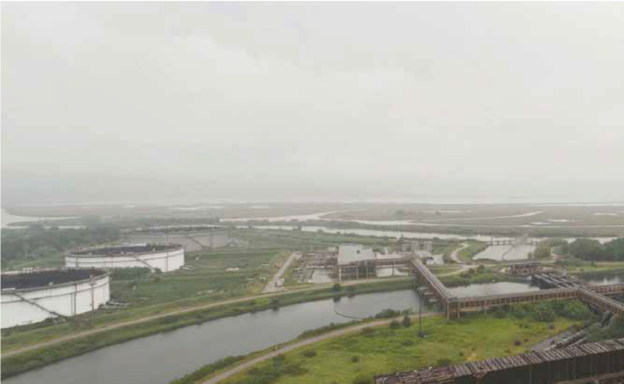
Fig. 229 Oil tanks and water adduction system (source: Enel)
