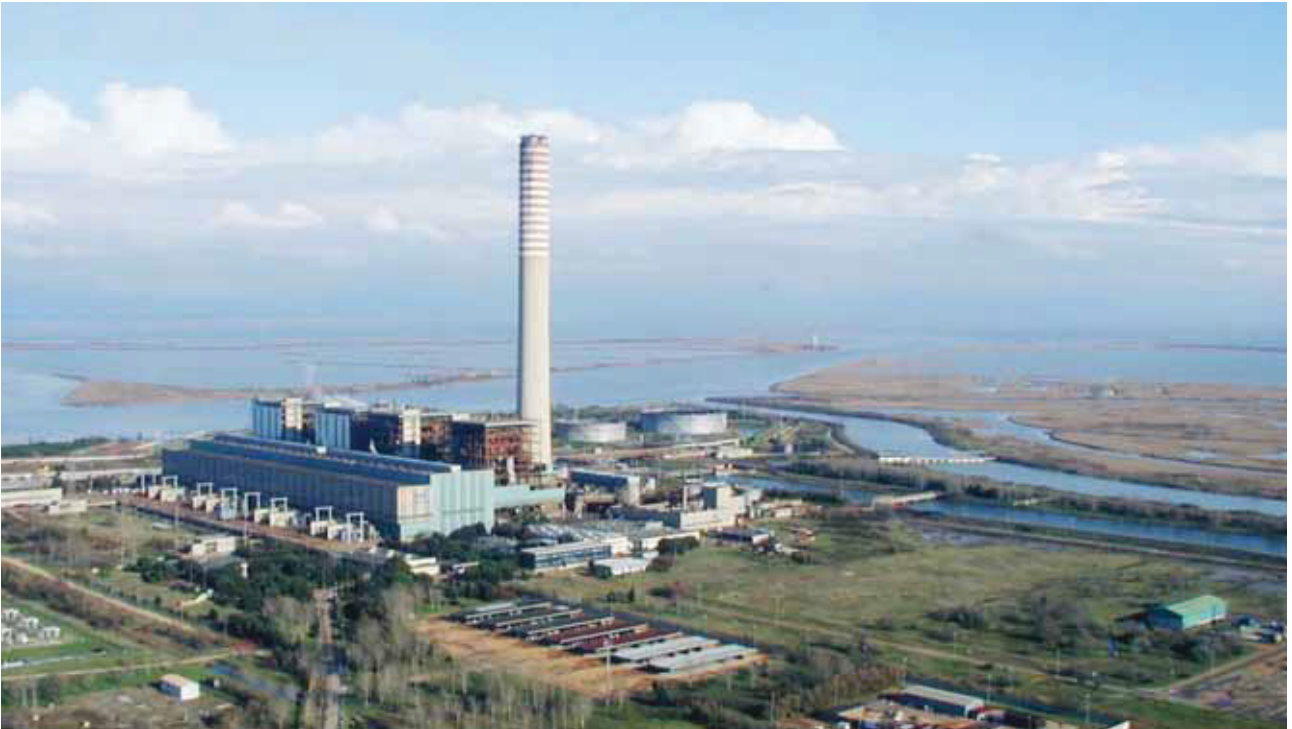
Fig. 223 The integration of the Polesine Camerini power plant in the delta landscape (source: Enel)
