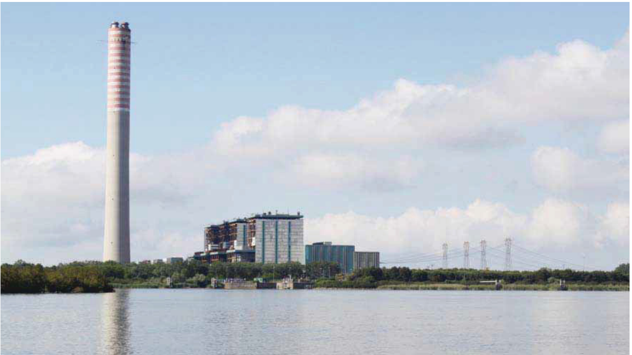
Fig. 224 The chimney of 250 m high (source: Enel)
