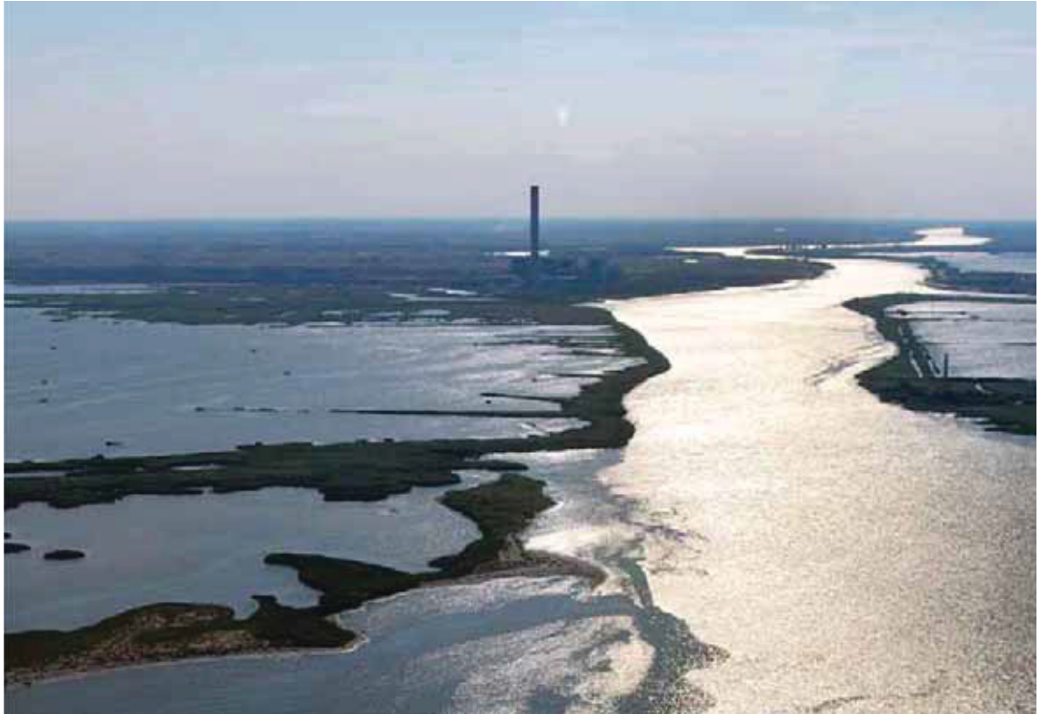
Fig. 201 The Po delta river and the power plant in Polesine Camerini (source: Quaglia)
