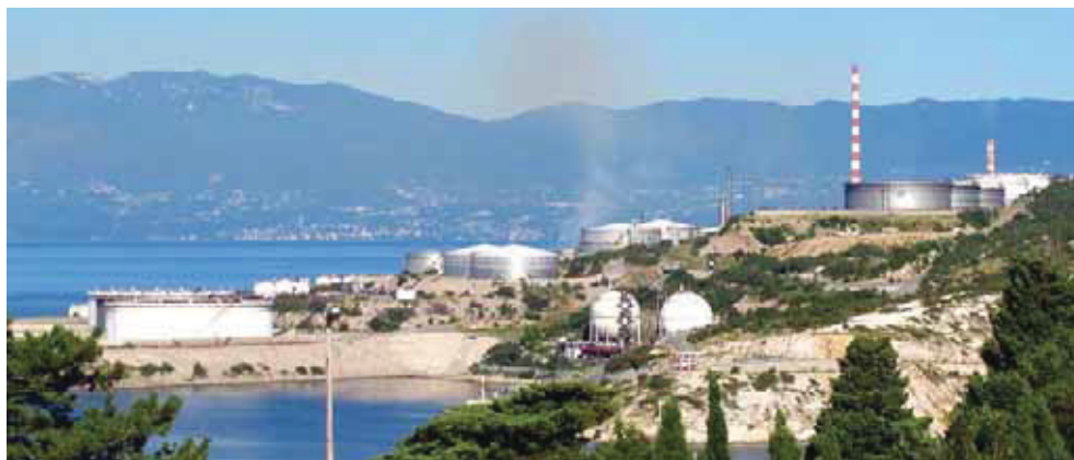
Fig. 64 MOL Rijeka oil refinery (source: https://commons.wikimedia.org/wiki/File:Kraljevica_2010_0728_02.JPG )
