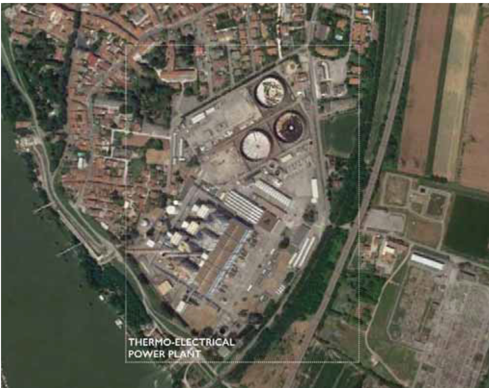
Fig. 185 Ostiglia thermal power plant (source: Bing Maps)
