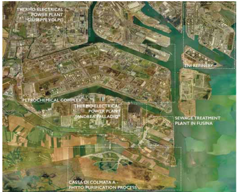
Fig. 179 Porto Marghera industrial harbour (source: Bing Maps)
