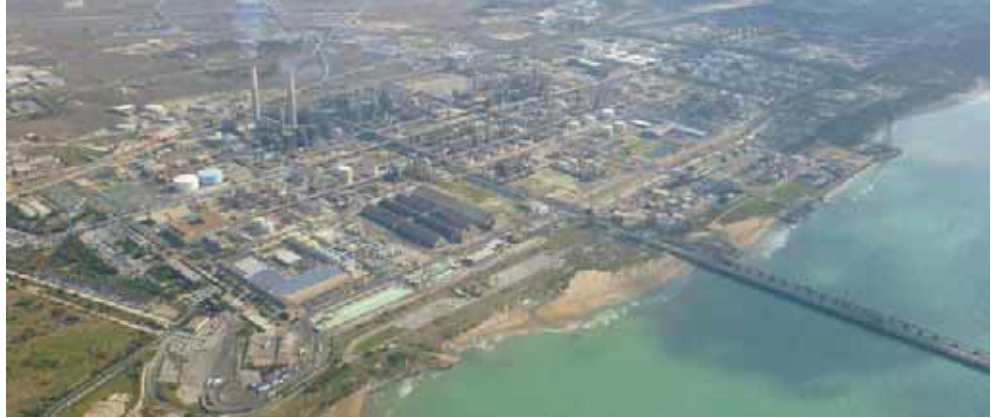
Fig. 60 ENI Gela refinery (source: https://commons.wikimedia.org/wiki/File:Gela_zona_industriale_dall%27alto.JPG )
