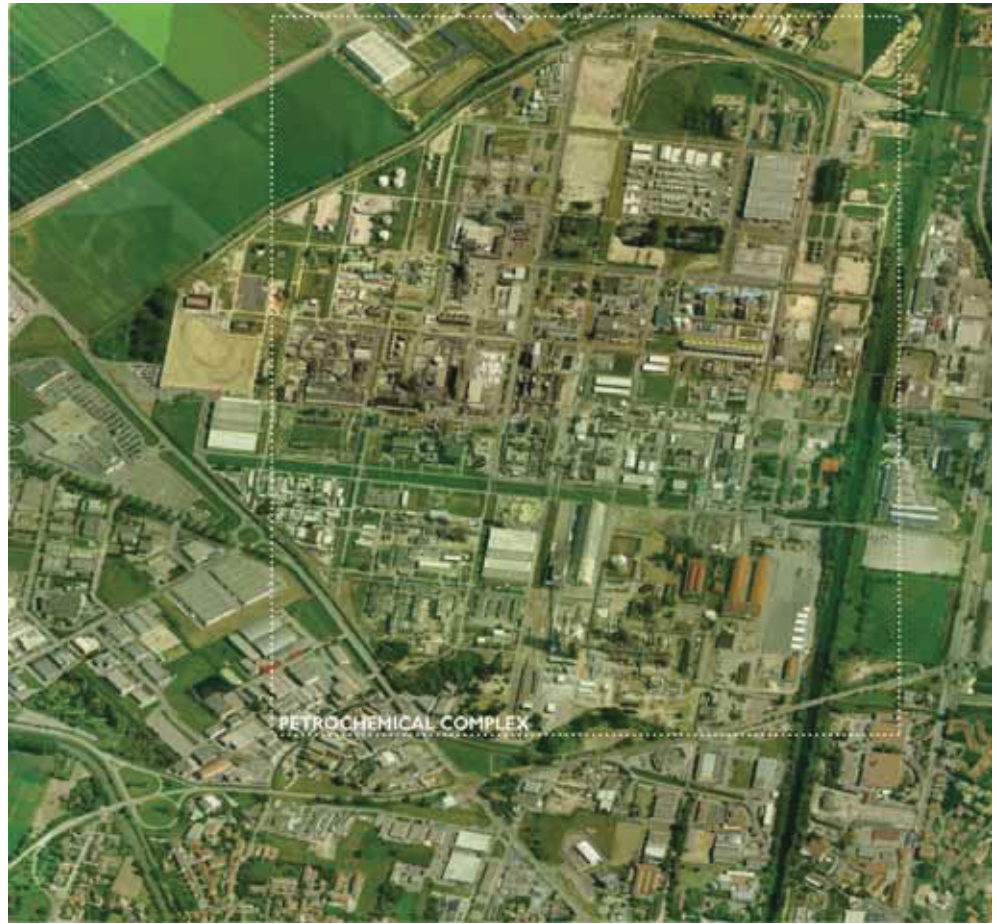
Fig. 182 Ferrara petrochemical plant (source: Bing Maps)
