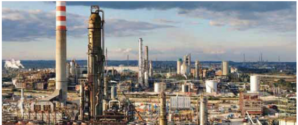
Fig. 62 Priolo Gargallo refinery (source: http://siracusa.gds.it )
