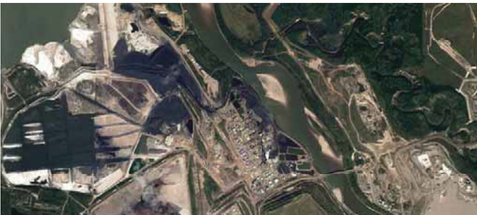
Fig. 37 Fort McMurray tar sands, Alberta, Canada, altitude: 8 km (source: Google Earth 2017)
