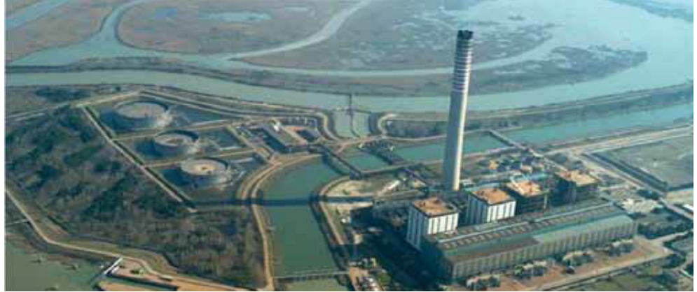
Fig. 52 ENEL Polesine Camerini power plant (source: http://www.bioecogeo.com/33206-2/ )
