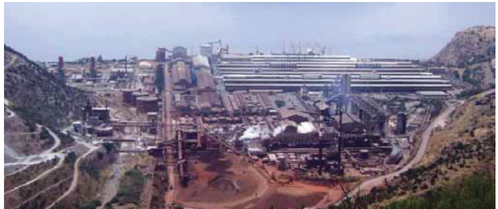
Fig. 74 Agios Nikolaos power plant and aluminium industry (source: http://www.stager.gr/index.php/gr/works )
