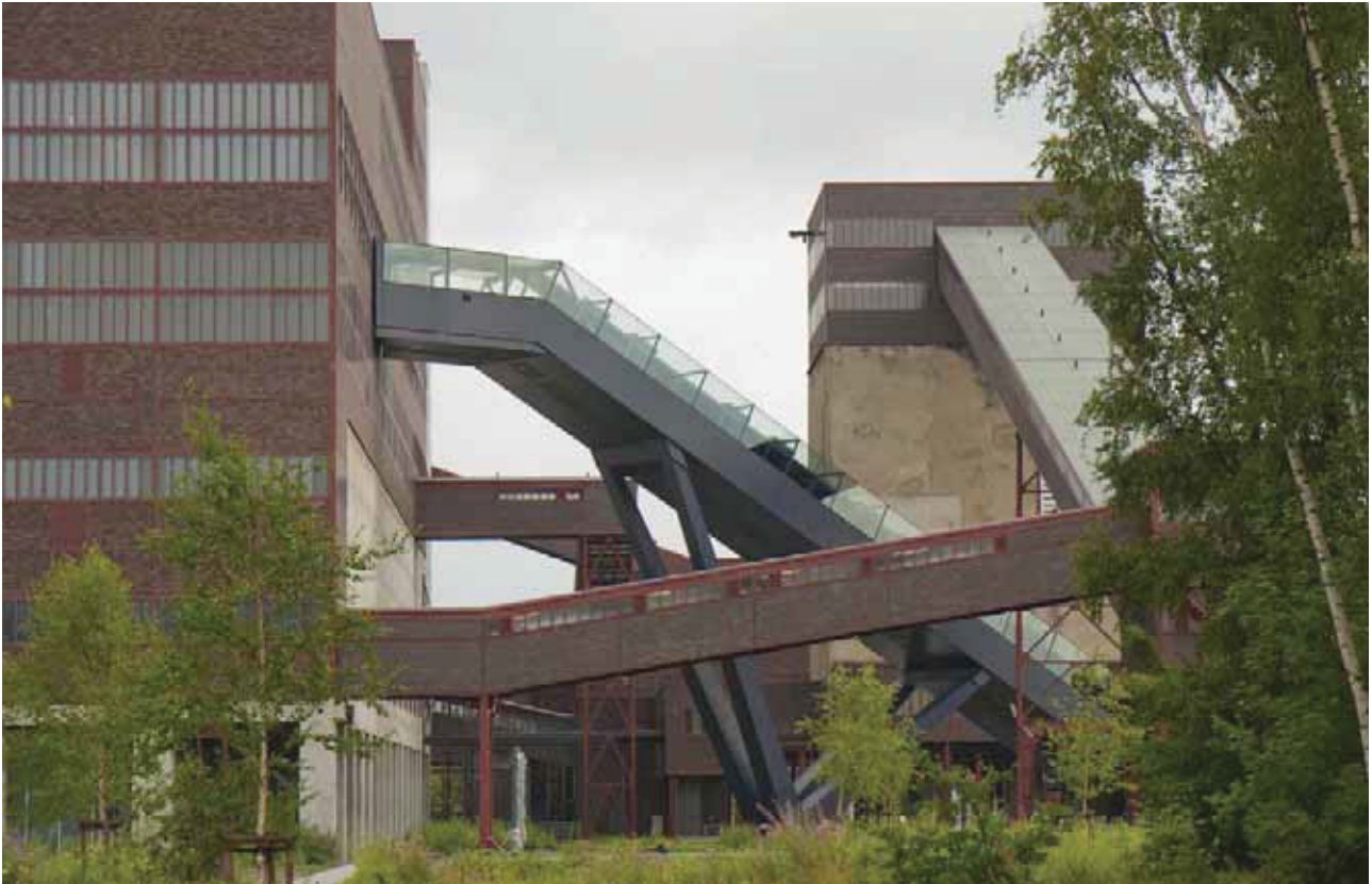
Fig. 117 Entrance to the Ruhr Museum realized by OMA (source: Anselm Van Sintfliet)
