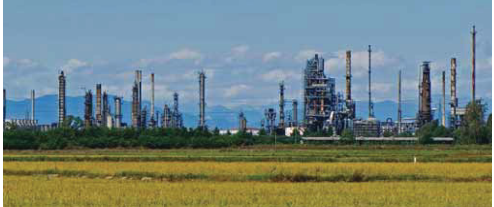
Fig. 48 Exxon Mobil-ERG Trecate oil refinery (source: www.antonini-foto.it )
