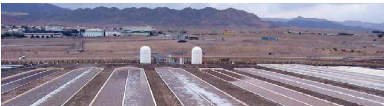
Fig. 169 D-FACTORY project: open raceway ponds (source: D-FACTORY project)
