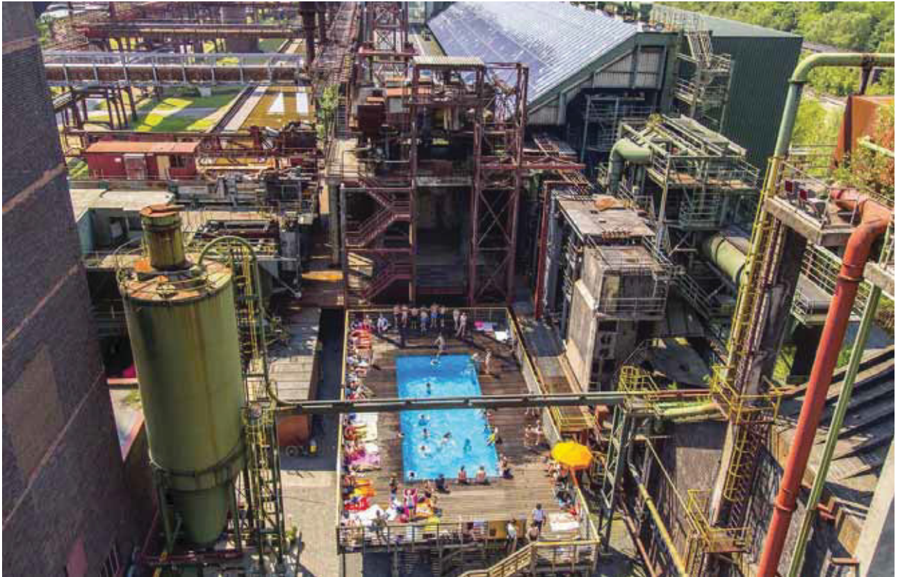
Fig. 119 Pool in Kokerei plant (source: Jochen Tack)
