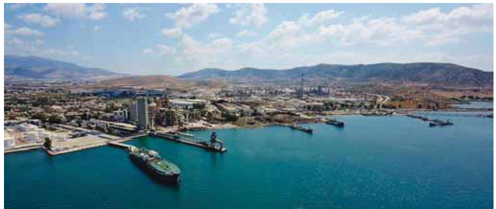
Fig. 75 Aspropyrgos refinery (source: https://www.tripinview.com/en/places/residential/55736/greece-attica-central-attica-aspropyrgos )
