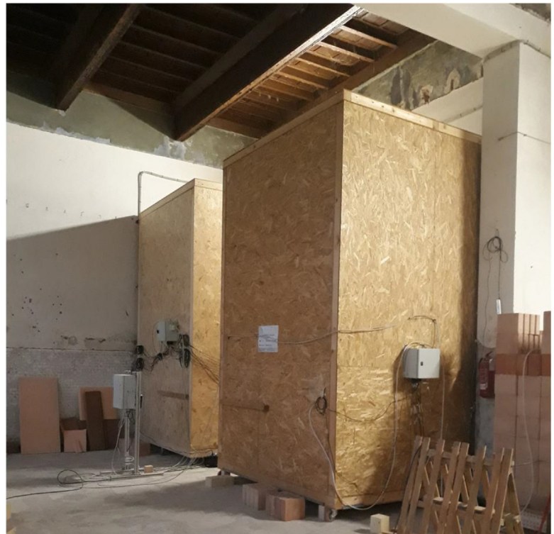
Fig. 5. a) Positions of the two metering hot boxes and the insulation technologies, b) The two metering boxes in the test room.
