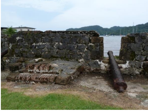
Figure 1.2.1.8. Inner view of sea-front walls of Fort San Jeronimo. Picture took in the beginning of September 2014 at 12:00 a.m.
