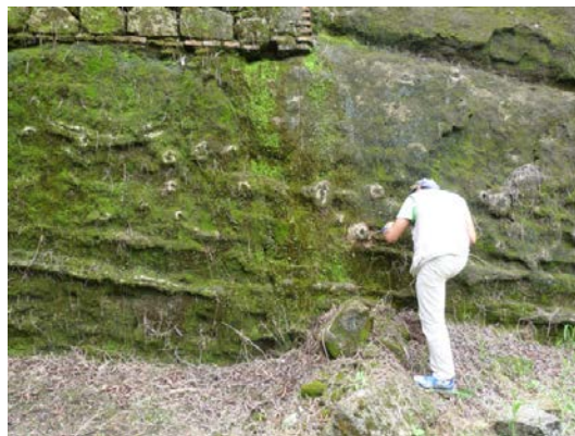
Figure 2.1.3. 7. Outcrop of sandstone/tuffite forming the bastion foundation.
