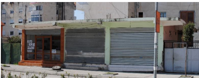
Attached, non-residential buildings, with no style
