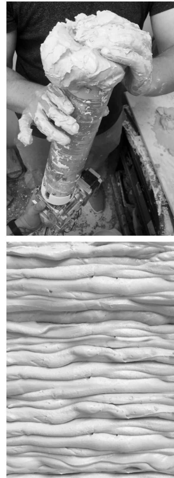
Fig. 7.35 Above: manual filling of the tube containing the extrusion material. This process can be improved by using mechanical systems for filling that prevent the formation of air bubbles in the liquid-viscous mixture. Below: resolution of the extruded layers that define the volume of the gap. The presence of inaccuracies and air bubbles can be improved and depends partly on how the container is filled.
