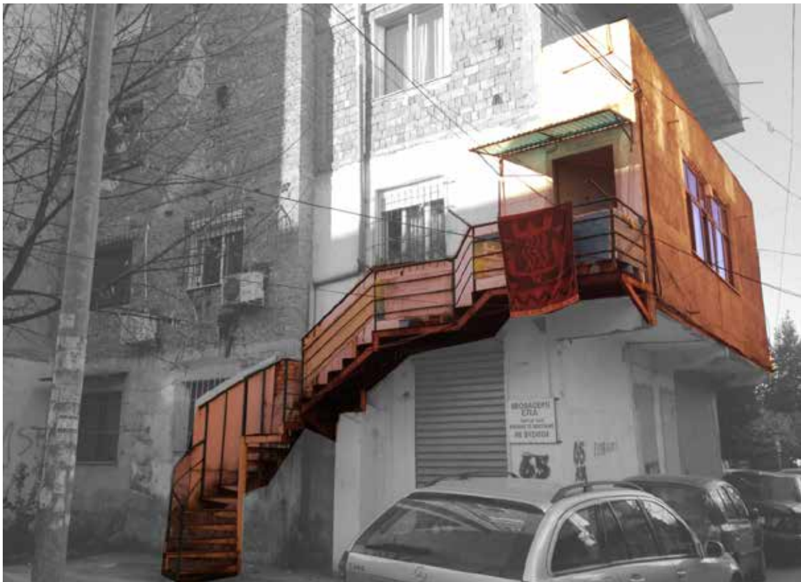
Figure 8-8. “Continuity and discontinuity of individualization of the society”. Occupation of an abandoned public surface by private access stairs to a multi-dwelling building. Source: author.
