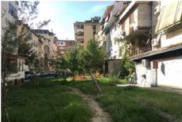
COURT_LANDS - abandoned playground
