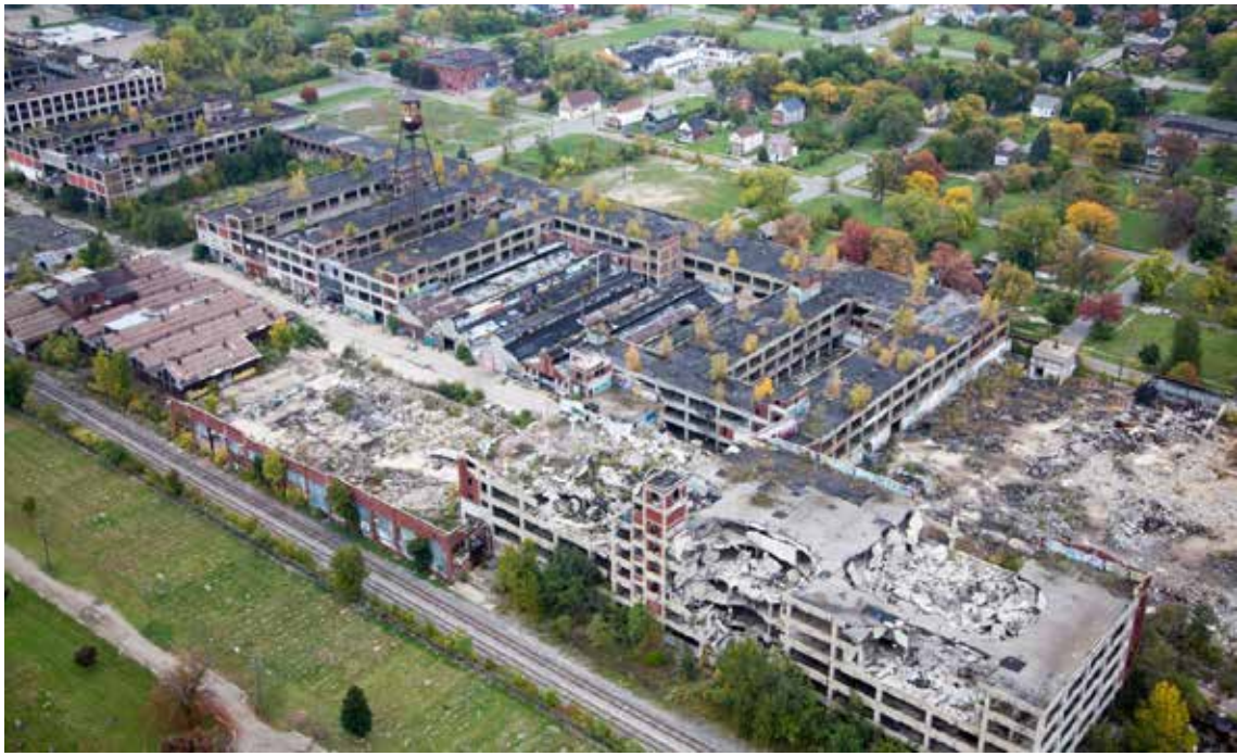
Figure 7-23. The Packard plant, regarded as a sophisticated auto production facility when it opened in the early 1900s, now in ruins. Source: Photographs by Alex S. MacLean. https://www.nytimes.com/interactive/2014/12/07/opinion/sunday/exposures-detroit-by-air-alex-maclean.html
