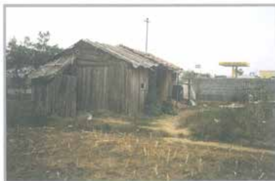
Building a "barrake"
