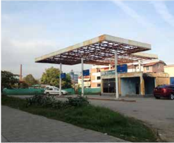
INFRA_LANDS - abandoned gas station
