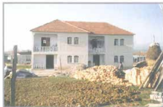
Completing the house
