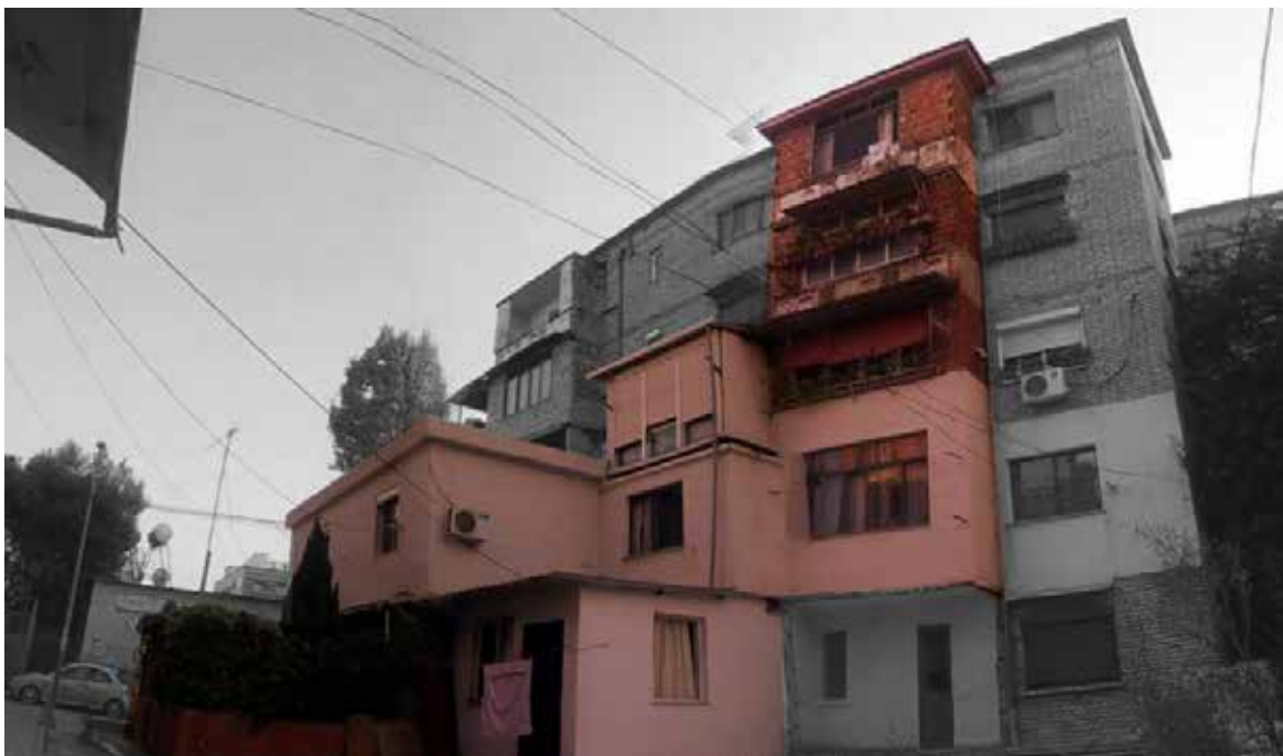
Figure 8-9. Illegal additions to existing buildings: floor additions, illegal buildings in private or public land for business (in the city centre) or housing purposes (in city outskirts). Source: author.
