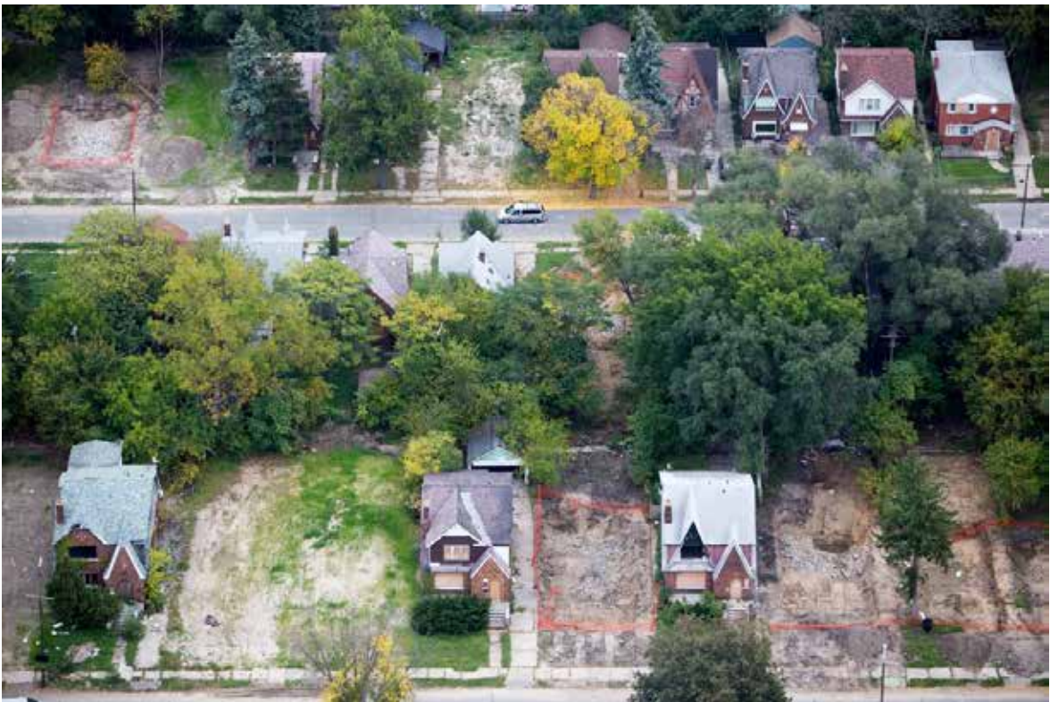
Figure 7-22. Lots of recently demolished homes overgrown with vegetation in the Fitzgerald neighborhood of Detroit. Source: Photographs by Alex S. MacLean.
