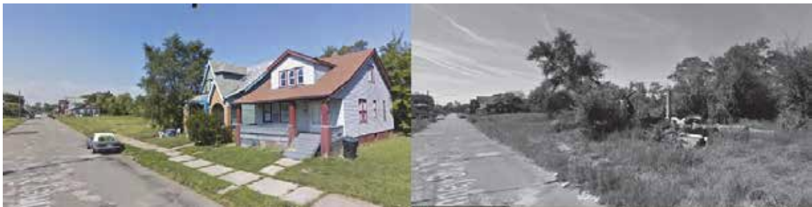
Figure 7-24. Abandoned and demolished houses in Detroit. Source: http://www.urbanmarkers.ro/actions/how-to-perceive-the-importance-of-small-scale-actions-in-a-big-scale-perspective/
