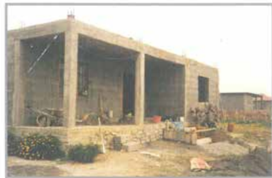
Building the first floor
