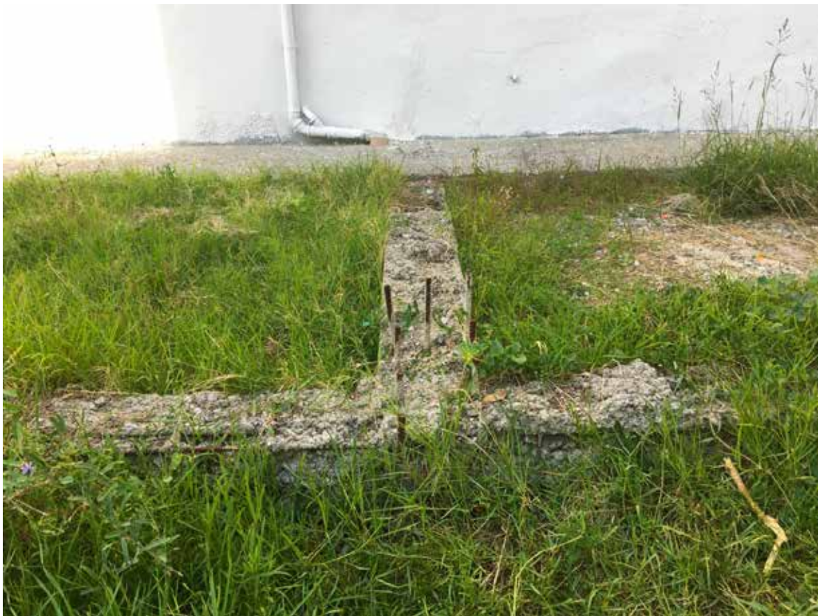
Figure 8-15. Demolished building ruins in a Residual Landscape, Tirana. Source: author.
