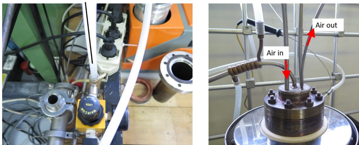
Figure 4.50: Compressed air flange cooling
