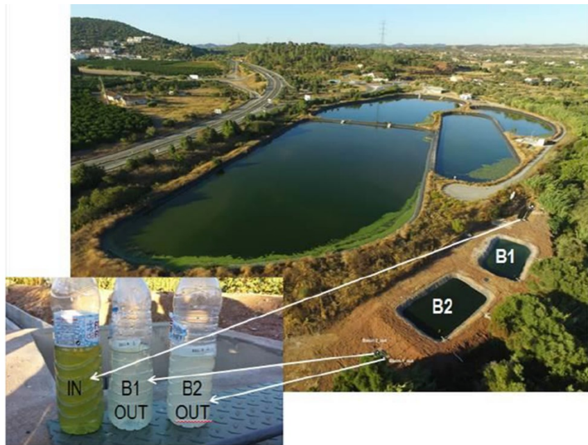
Figure 50. Soil column experiments and infiltration basins in Algarve (Portugal) at the Wastewater Treatment Plant.
