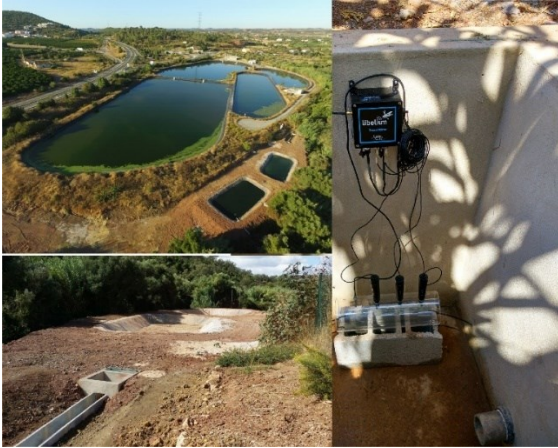
Fig 8. MARSOL SAT basins at São Bartolomeu de Messines waste water treatment plant (South Portugal) [41].
