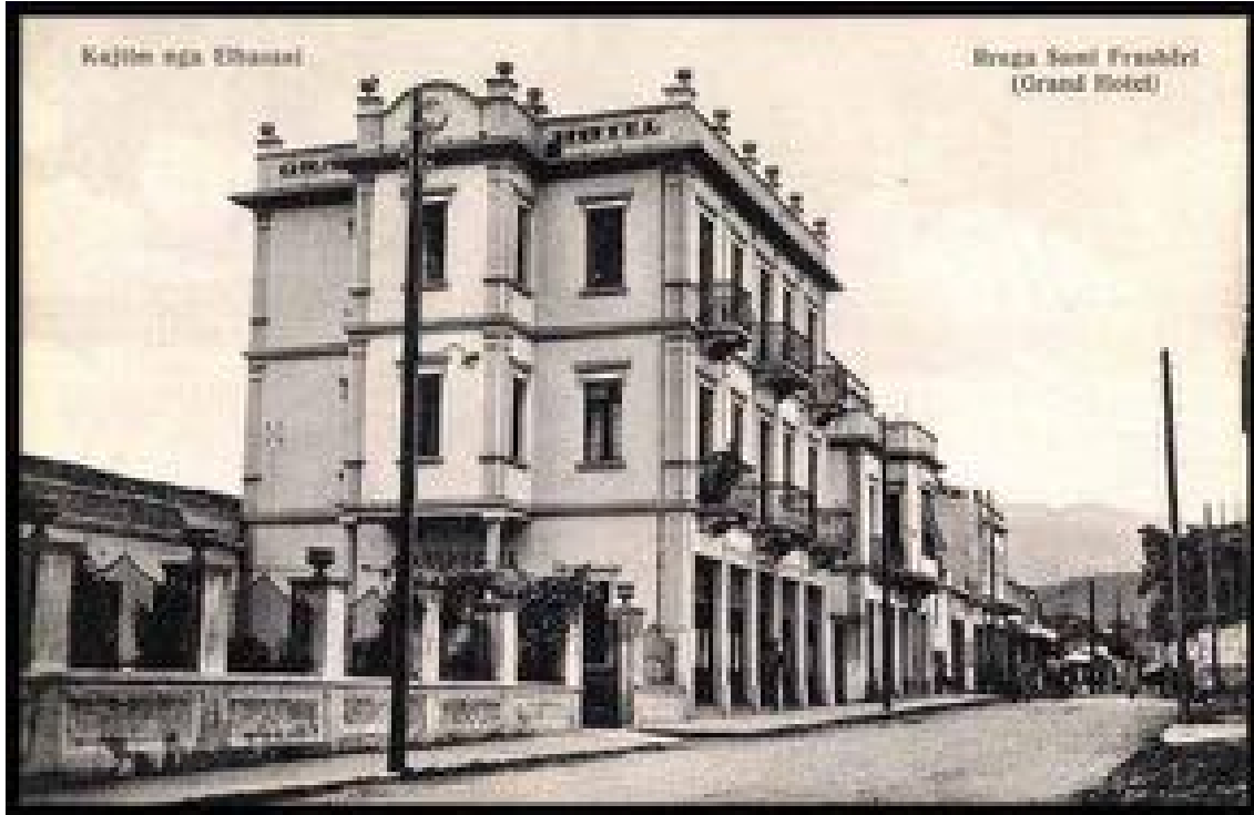
Figure 4.28 "Grand Hotel (Ish- turizmi I vjeter) dhe rruga qe me pare quhej Sami Frasheri, sic dukeshin ne vitin 1938" in Elbasan, in an old postcard, 1938 (source: ElbasaniAD archive, donation of Fiqiri Drinziu)
