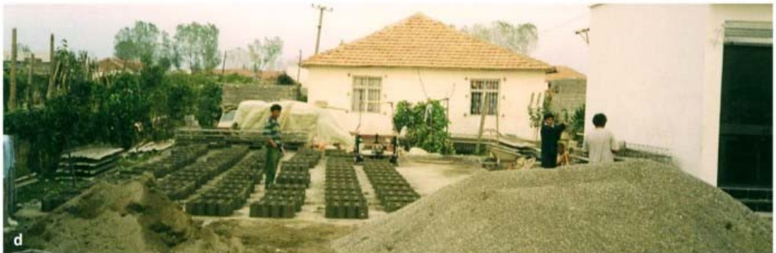
4.63 Typical rural “family houses”; built through the help of the “master builders” with self-made cement blocks produced in the area, or by families themselves (source Co-PLAN archive)
