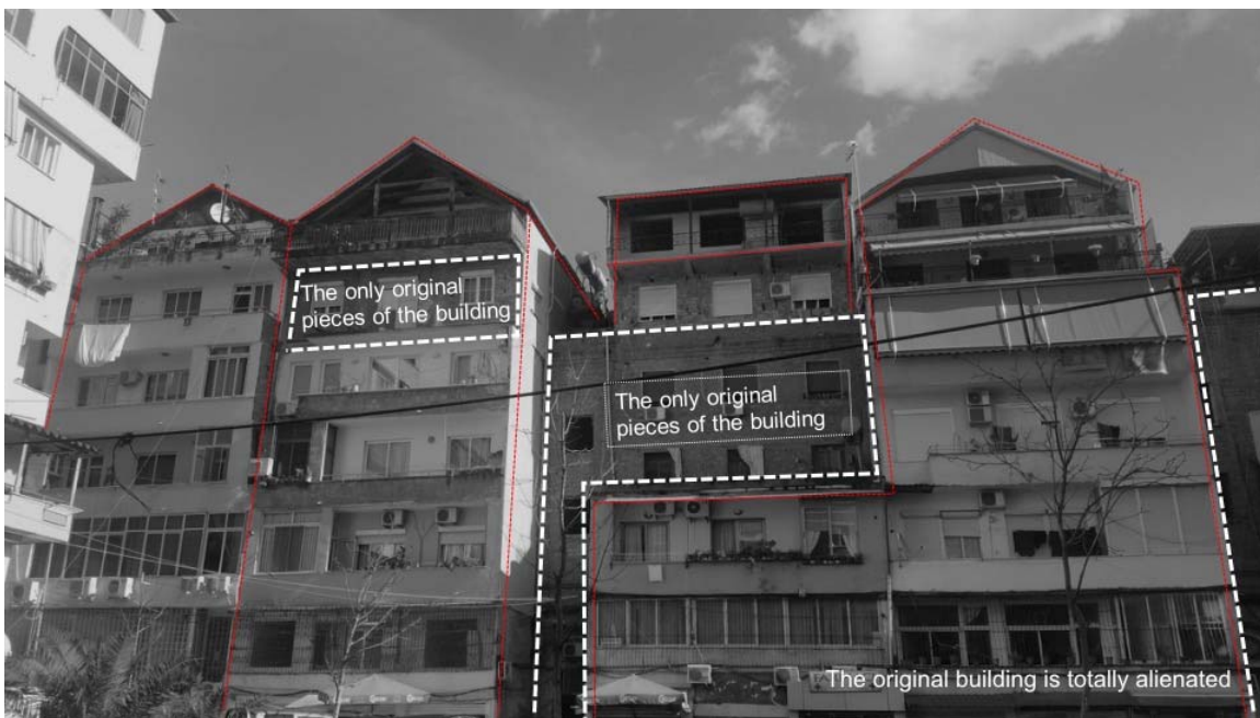
4.50 Recording Over space-occupiers: fill-in; and parasite-ing structures in relation to the frames; (pictures from the analyzed samples)
