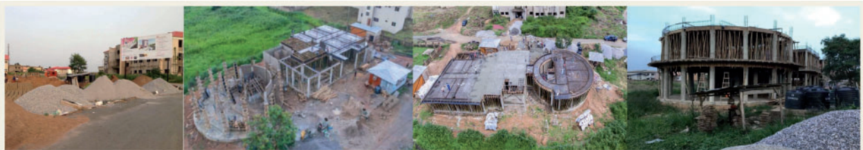
Figure 7 EHC Centre construction in Ibadan, Nigeria.
