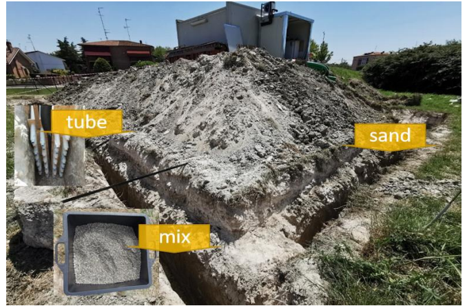
(e) Trenches of the geothermal closed loop
