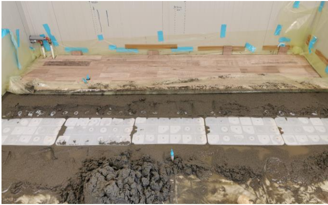
(a) Installation of the radiant floor
