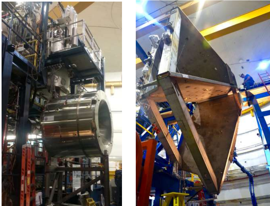
Figure 4: The CLAS12 magnet systems. Left: The fully assembled solenoid magnet including all cryogenic connections on the beamline at the beginning of cool down, before the detector installation. Right: The torus magnet with all six coils mechanically assembled in a common cryostat. The coil cryostat, which is fabricated from non-magnetic steel, has an outside width of 124 mm. The cross bars provide a cold (4.5 K) cryogenic connection of neighboring coils, and counteract the out-of-plane forces to provide mechanical stability to the full magnet. Due to the large physical size of the assembled torus magnet, the final assembly of the magnet had to be completed in Hall B.
