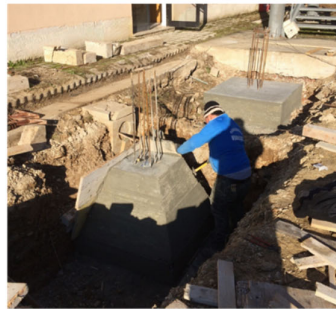
Figure 1. Sketch of the RC frame realized at the Hydrogeosite Laboratory (a,b): the structure is constituted by two columns (C1 and C2) and two beams (B1 and B2). Two different types of foundations are realized (F1 and F2). Photos of an intermediate constructive phase (c) and the final construction (d).
