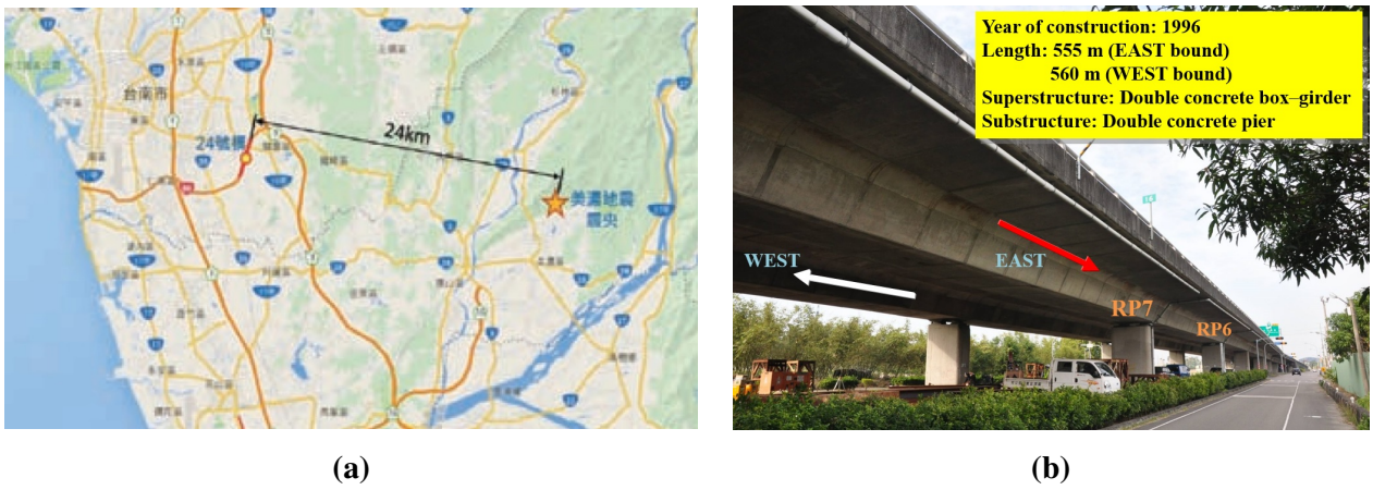
Fig. 8. (a) Location of “2016 Southern Taiwan earthquake”. (b) Bridge No. 24 of Highway No. 86, Taiwan.
