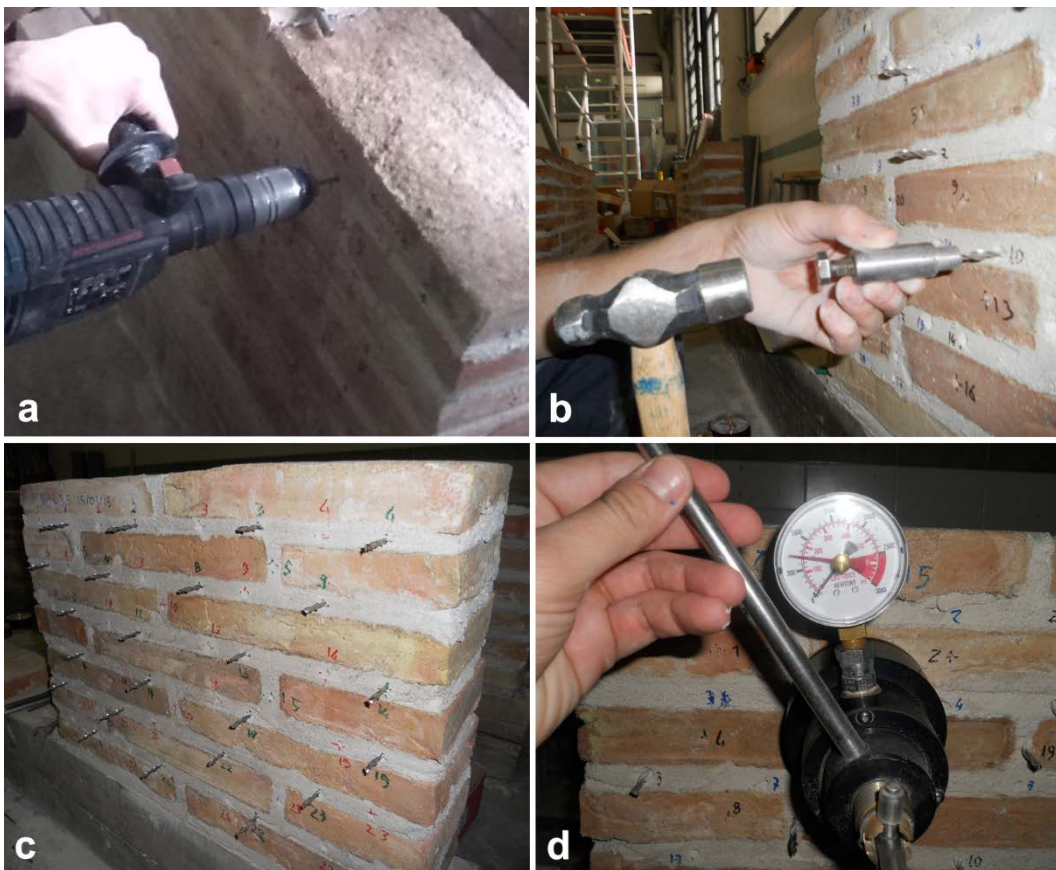
Figure 6 – Operation of the screw (helix) pull-out test: drilling the pilot hole (a), insertion of the helix into the bed joint using the sleeved driving tool (b), helical ties ready for extraction (c) and pull-out with the loading device (d).
