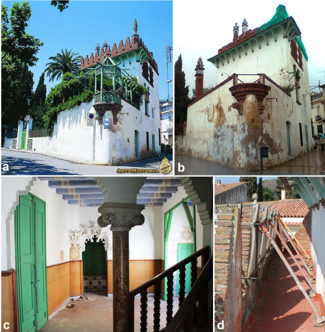
Figure 10 – Casa Puig i Cadafalch in Argentera, Barcelona: exterior view before (a, copyright ArteHistoria) and after the collapse of the pavilion and the merlons (b), view of the interior (c) and emergency propping of deformed merlons (d).
