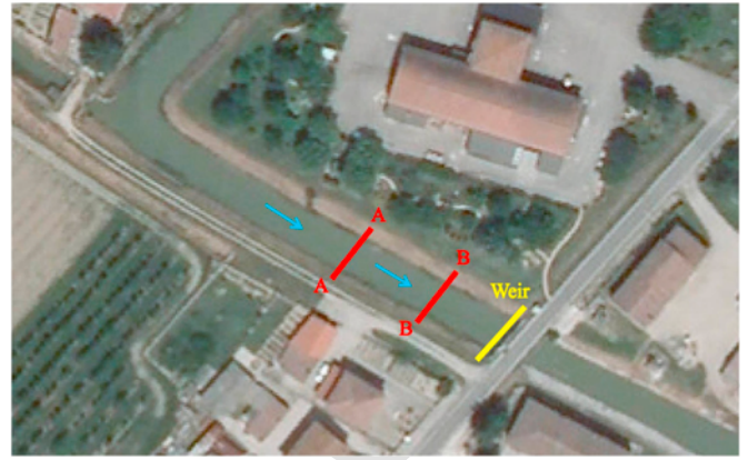
Fig. 2. Location of the investigated cross section along the Fossa Masi channel.
