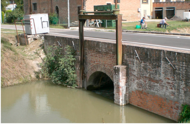
Fig. 4. The downstream weir along Fossa Masi channel.
