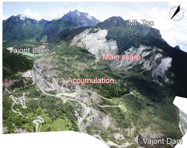
Fig. 7 - Drone photo of the main landslide body.
