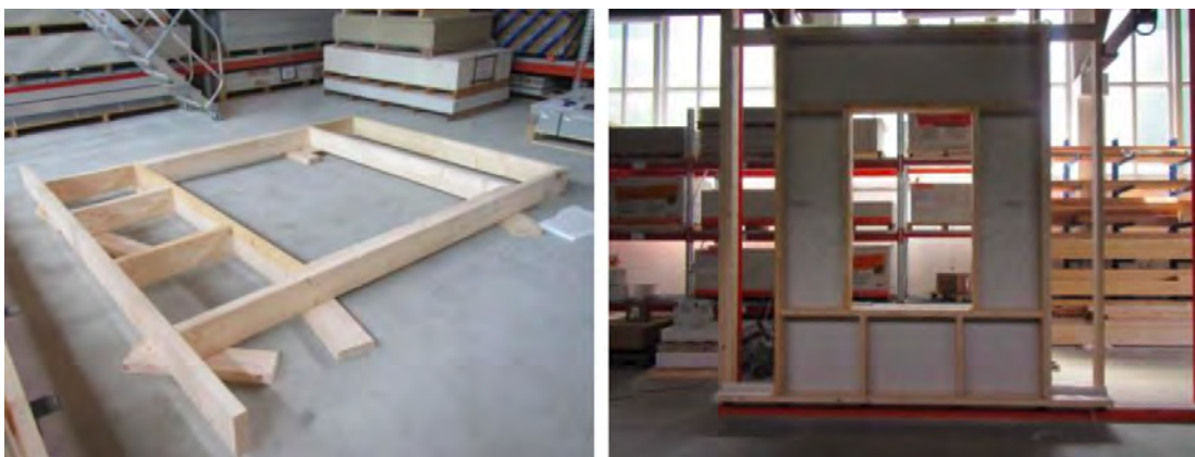
Figure 2. Example of PnP building component: multifunctional façade panel constructed by Fermacell
