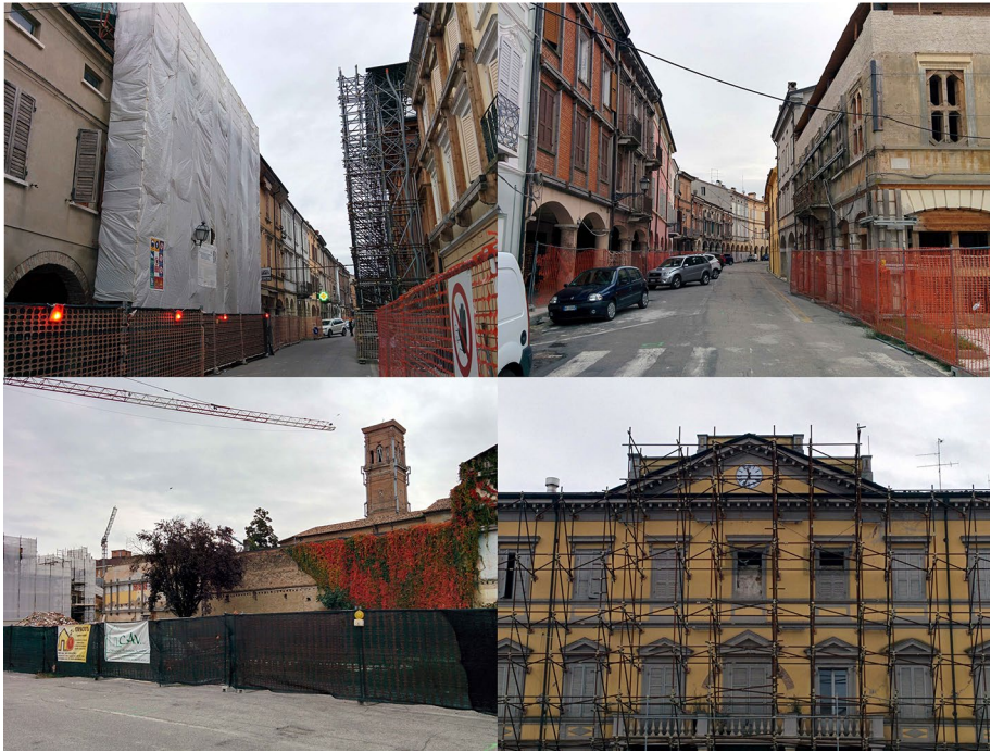
Fig. 2 Damage after the 2012 NIE in the Concordia sulla Secchia city centre. Pictures taken on May 29th, 2016, 4th anniversary of the earthquake
