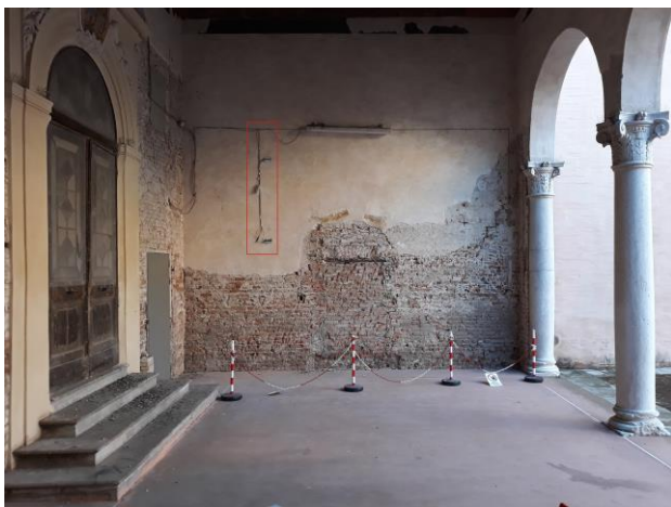
Fig. 2. Outdoor picture of the studied wall (located in Palazzo Tassoni internal courtyard, under a porch) [26].
