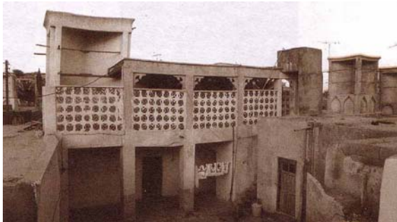
Figure 3- Taremi is perforated screen used in portico
