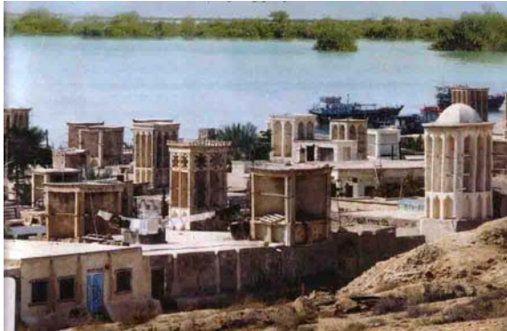
Figure 8- Wind towers of hot and humid region are usually larger than the ones in hot and arid region.
