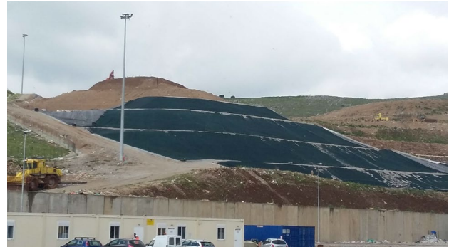
Figure 3. HDPE used as cap for the sector #1 and sector #2 of the landfill #6 (from RAP S.p.A. website).
