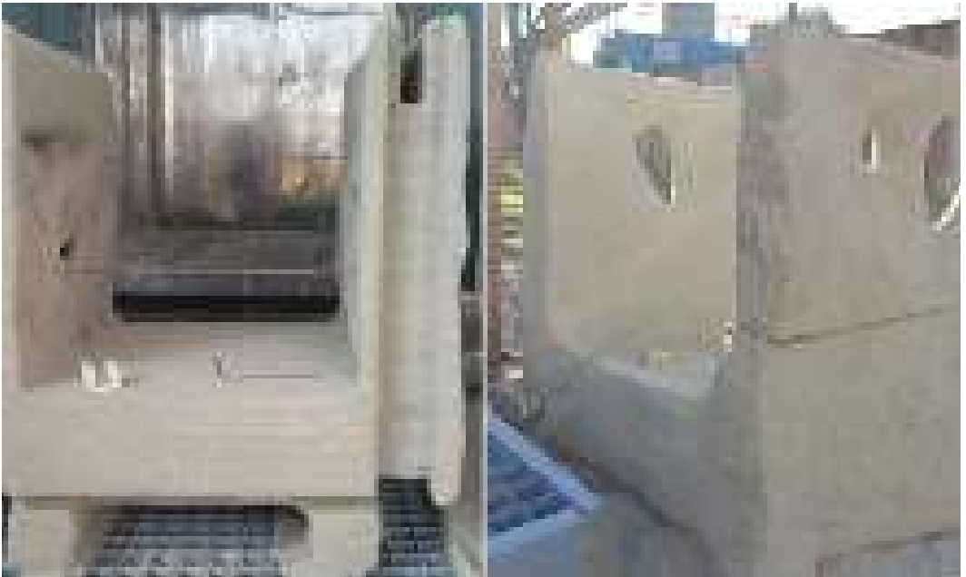
Fig5 / Sections of the 3D printed pedestrian bridge. The organic-shaped volume follows forms of nature with the aim of optimising the mechanical performances and the use of resources by recycling the raw material during manufacture source / photos of Dshape
