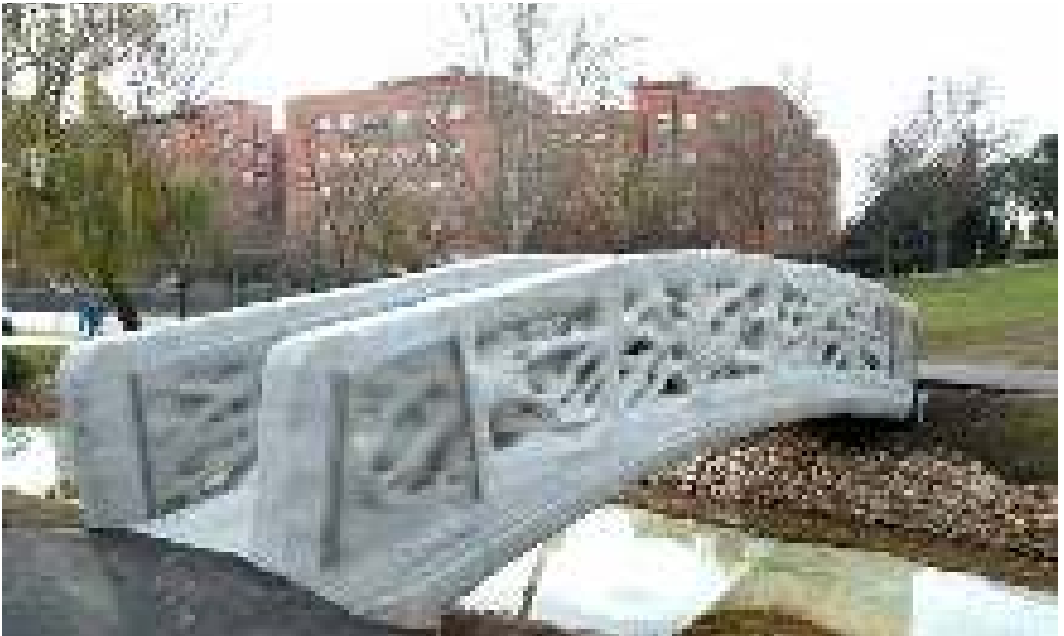
Fig4 / The 3D printed pedestrian bridge experimented in Madrid by Dshape and IAAC, through powder-bed deposit processing. It represents the first landscape component realised by the application of large-scale rapid prototyping. source / photos of Dshape
