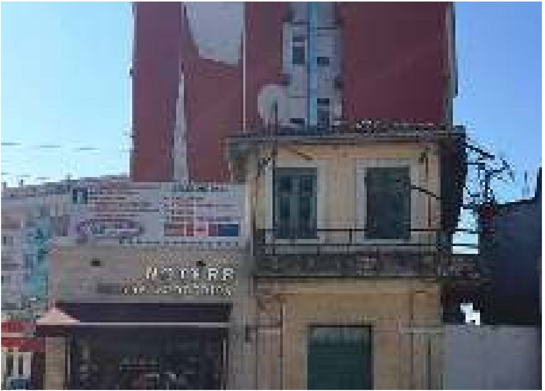
Fig4 / Existing housing stock in the inner city of Shkodra source / the author
