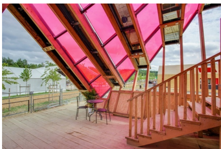
Fig. 6.2.3: Under the canopy the light gets a red hue caused by the re-emitted light that doesn't undergo total internal reflection
