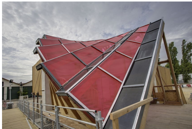
Fig. 6.2.4: Detail of the canopy: the panels were kept in place by aluminium profiles sealed with natural rubber gaskets while the wires ran inside the aluminium extrusions
