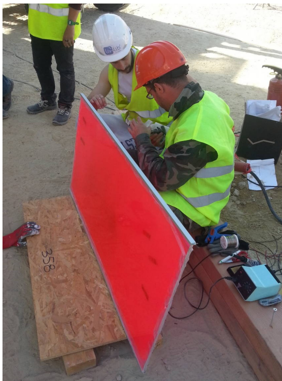
Fig. 6.3.4: A luminescent solar concentrator (LSC) module developed at Physics and Earth Sciences Department of University of Ferrara, the slab is still showing the protective film and the solar cells are enclosed in an aluminum profile
