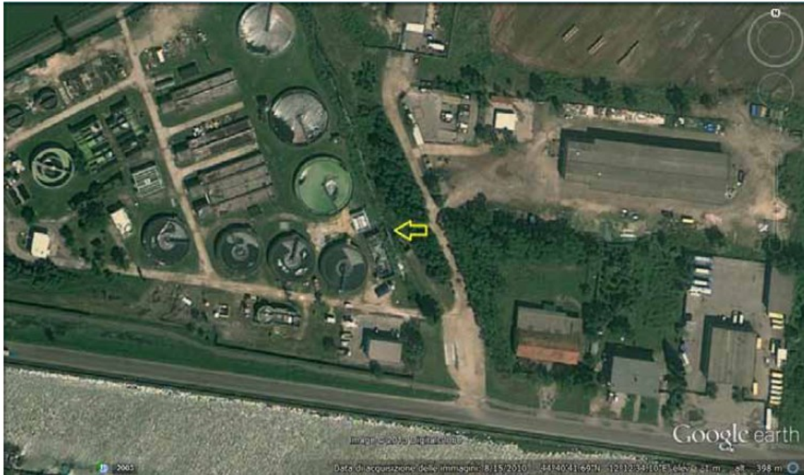
Fig. 8.7: Satellite image indicating the exit of the overflow upstream of the purifier MD
