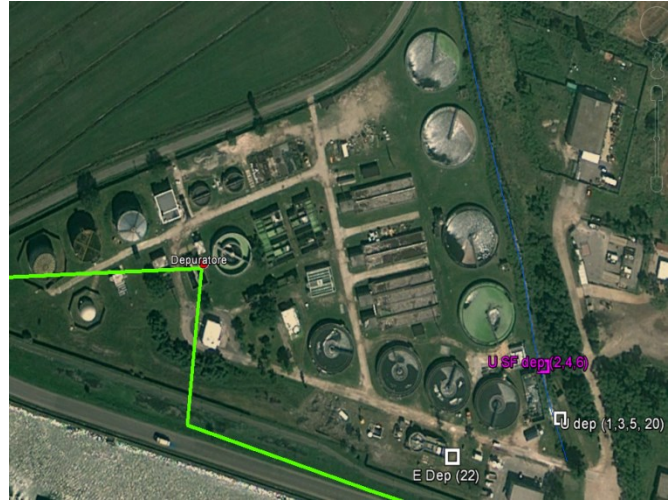
Fig. 8.17: View of the Comacchio WWTP, displaying the entry point (E Dep), the exit point into the canal Adige (U dep) and the upstream WWTP overflow (U SF dep).
