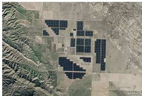
Figure 1.6. Satellite view of Topaz Solar Farm, a 550-megawatt photovoltaic power station made up of 9 million CdTe PV modules in San Luis Obispo County, California.
