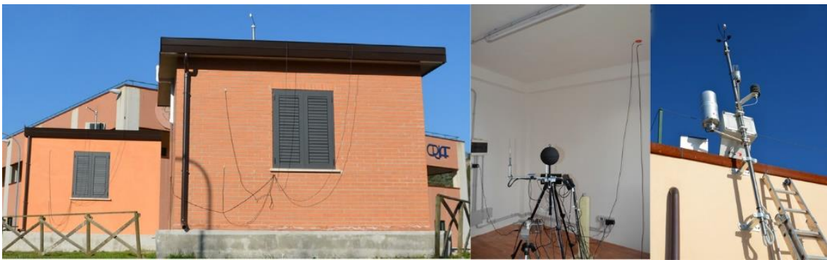
Figure 5.4: View of test-rooms and indoor–outdoor microclimate monitoring equipment [205].
