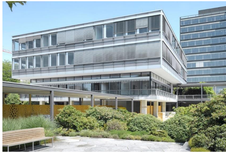
Figure 4.25: The renovation and refurbishment of building HPZ [186].
