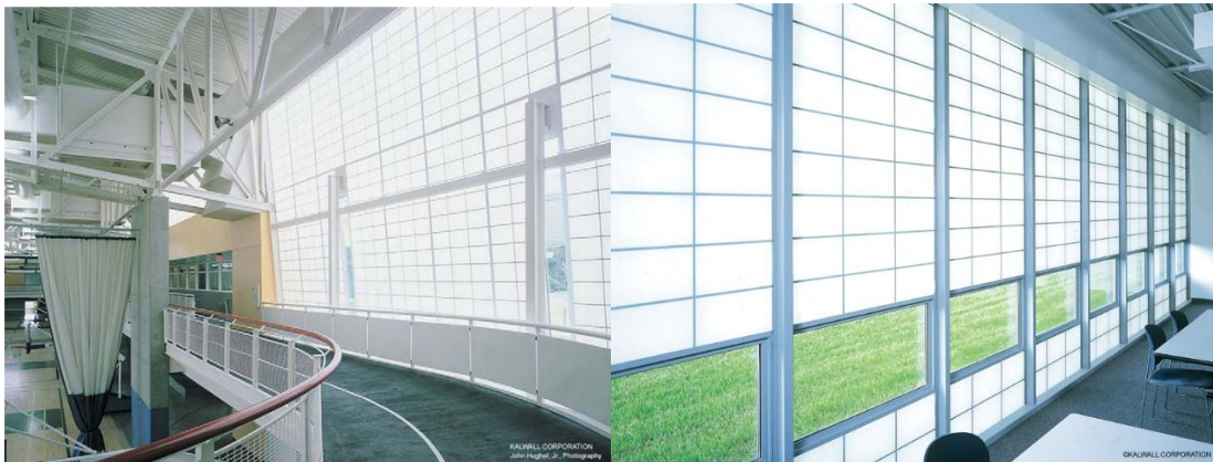
Figure 3.9: Examples of translucent aerogel for thermal insulation and daylighting [97].
