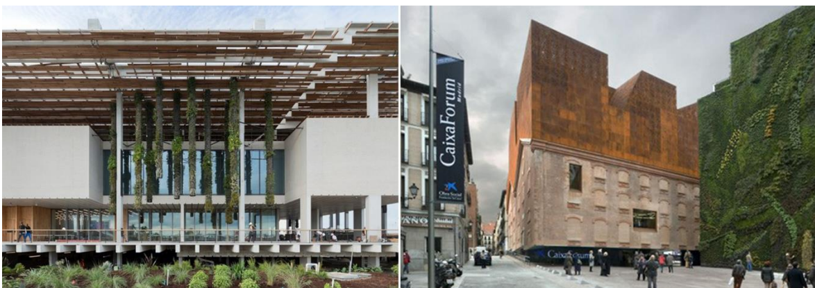
Figure 4.29: Two examples of sustainable development projects designed by Herzog & de Meuron, Pérez Art Museum Miami (left) and Caixa Forum, Madrid [194].
