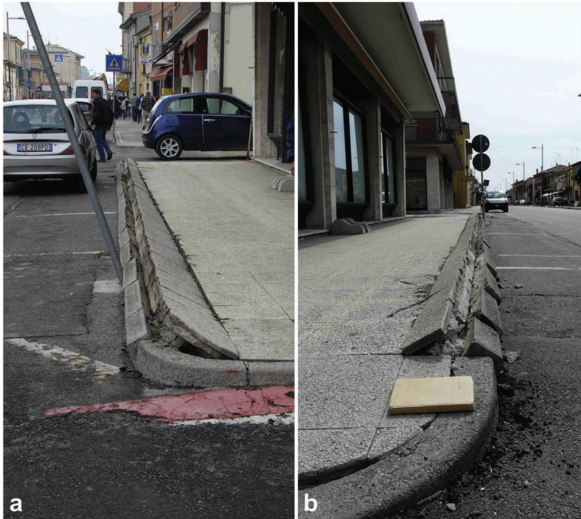
Figure 6.28: Example of an incipient buckling process affecting the top layer(s) and due to differential horizontal movements triggered by lateral spreading phenomena (from Papatthanassiou et al. , 2015).
