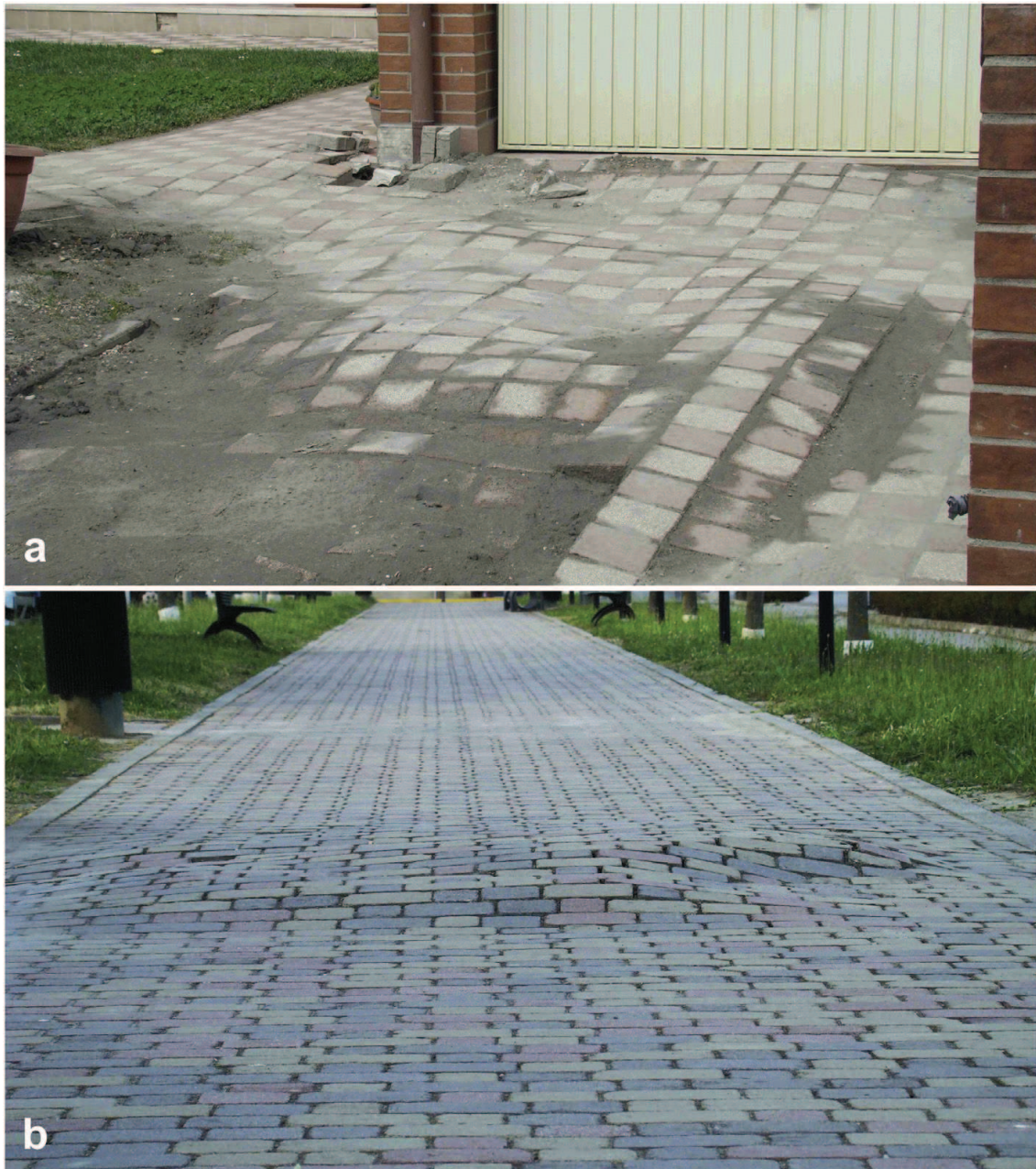
Figure 6.29: Examples of bulging phenomena caused by the failed attempt of sand ejection due to the presence of a strong cap layer (from Papathanassiou et al. , 2015).
