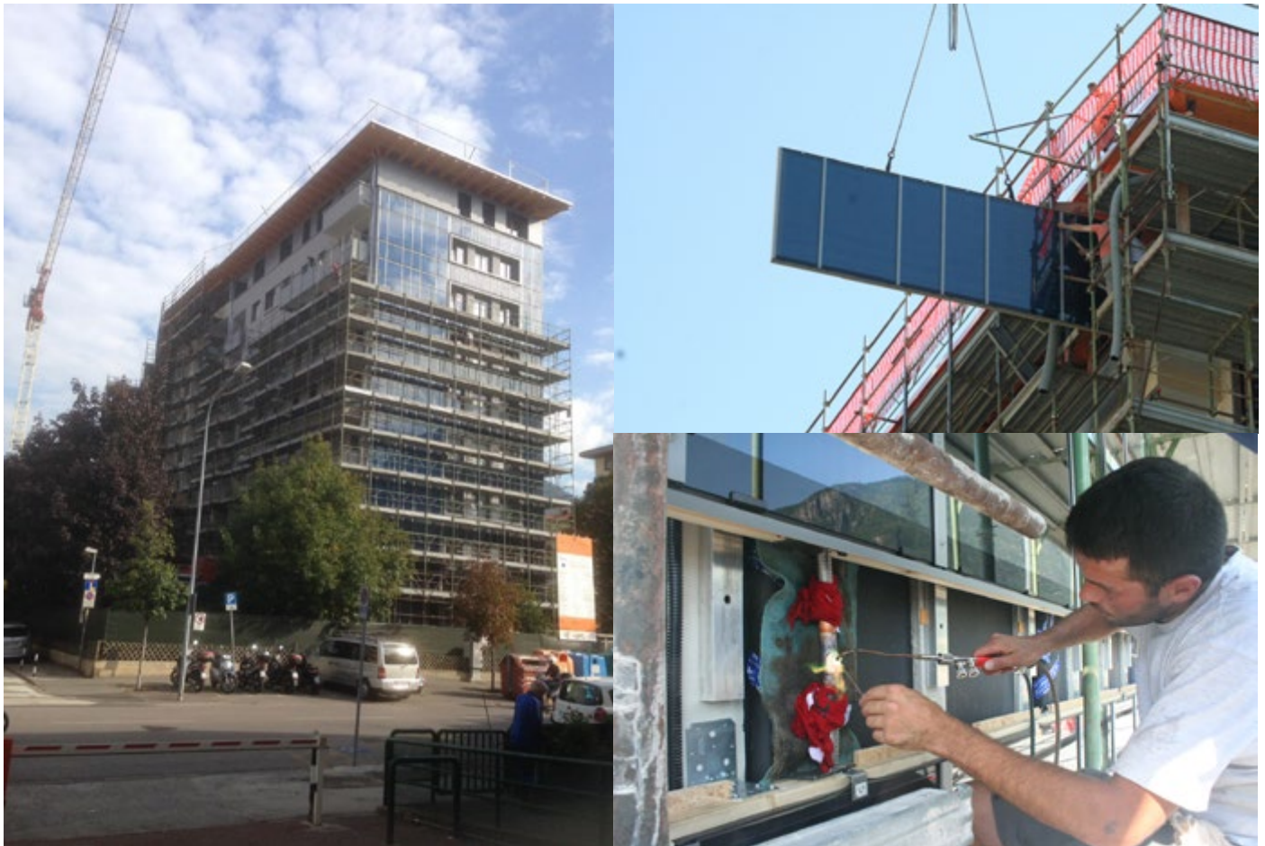
05 | Building works on the multipurpose façade in Via Brescia
