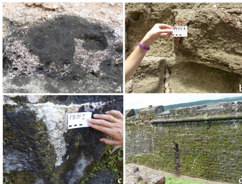
Figure 4. Pictures representing several deterioration processes observed at the sites. (a,b) at Panamá Viejo, (a) biological growth; (b) surface recession/material loss; (c) encrustation at Fort San Fernando (Portobelo); (d) biological growth at Fort San Lorenzo.
