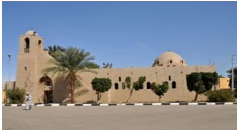
Figure 5.20 one of Hassan Fathy's high thermal mass mud brick buildings at New Gournah, Egypt
