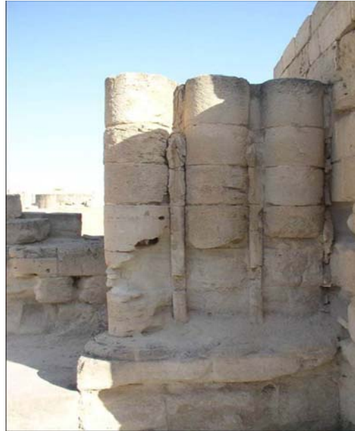
Figure 4.19: Deterioration of the sandstone of the Hisham's Palace
