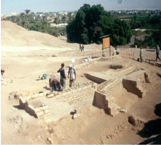
Figure 4.14: Building caps of new traditional mud-bricks on the ancient bricks in Tell es-Sultan
