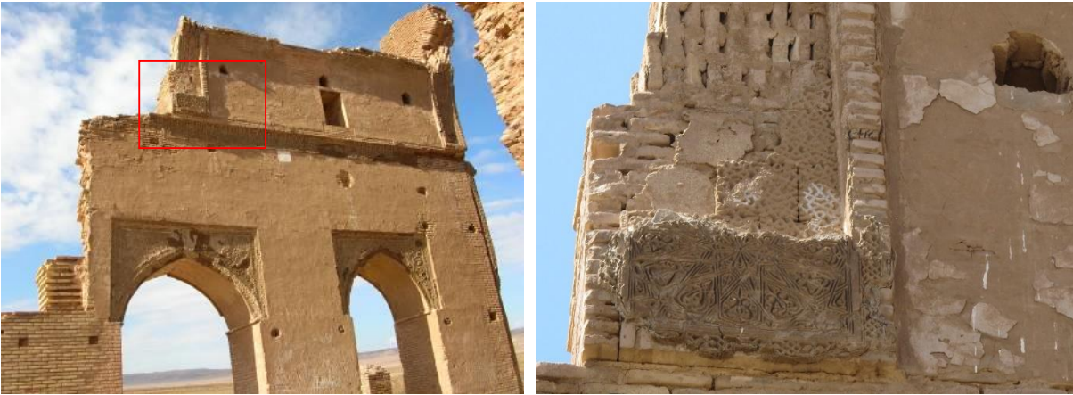
Figure 2.39. The location (left) and details (right) of the remaining pish-shekli bricks, covered by later stucco decoration at the Khosrowshir mosque
