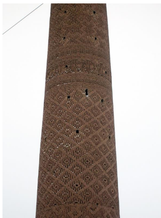
Figure 1.3. The Minaret of Khosrowgerd (1115 AD), arranged bricks and tarāshida elements in the decorative bands. (Unless otherwise stated, all photographs are by author.)
