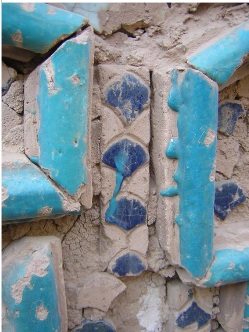
Figure 2.19. Applying dark-blue glaze on imbrication designs on a brick (inscription row of the back wall of the qibla iwan)
