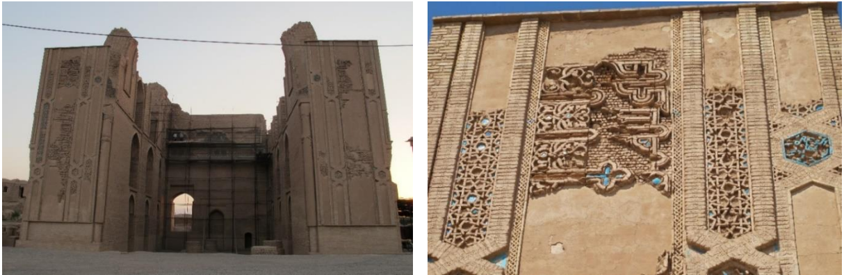
Figure 2.14. General view of the qibla iwan (left) and the interlacing bands, vertical sections and the decorations of the compartments on the façade of the qibla iwan (right) at the Zusan mosque.
