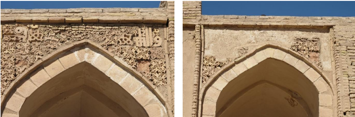
Figure 2.35. The spandrels of two iwanchas at the qibla side of the Masjed-e Sangān. The inserted elements at wrong place can be seen on the spandrel of the left hand iwan (left)
