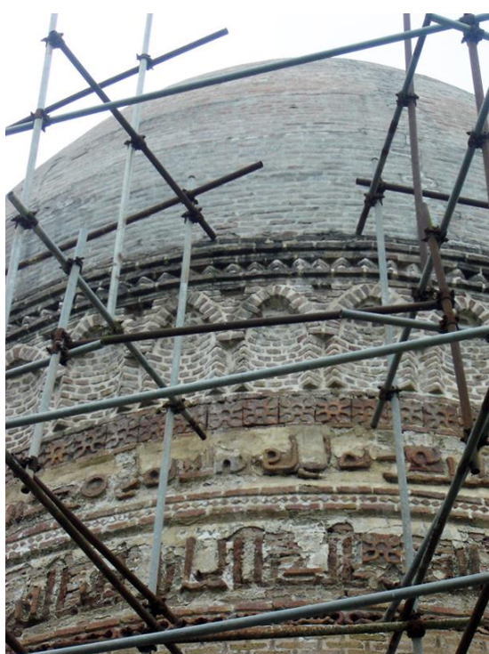
Figure 1.6. Borj-e Lājīm, patterns on top side of bricks together with arranged, borida and tarāshida elements
