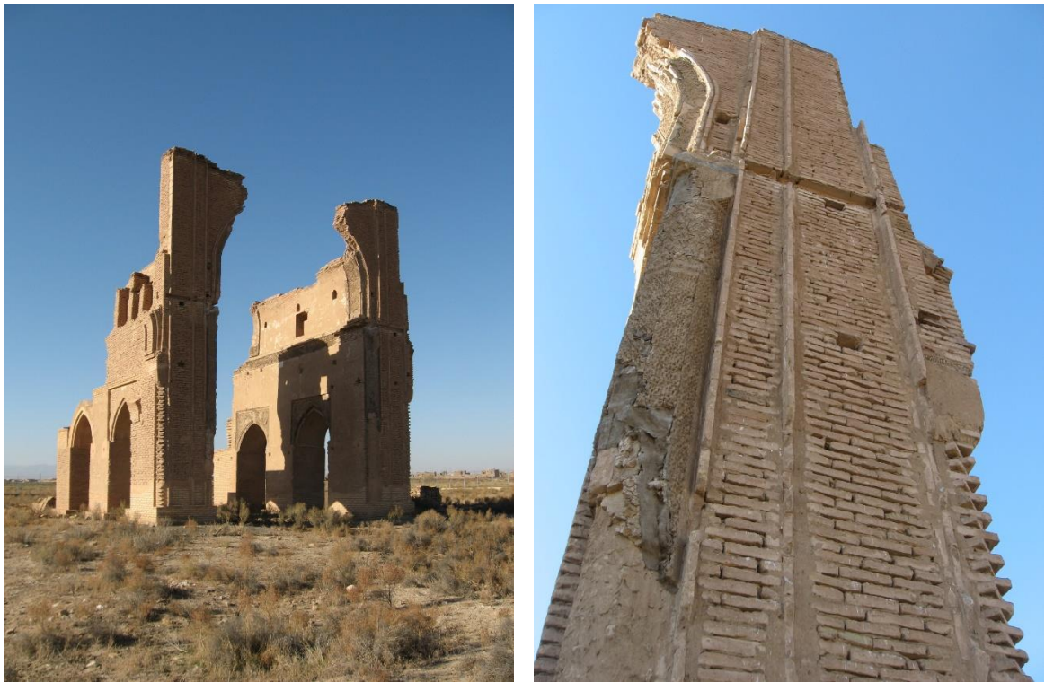
Figure 2.37. The east view of the Khosrowshir mosque (left) and the divided bands and decorative columns at the outer and inner edges of the iwan's façade (right)
