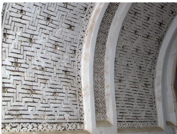
Figure 1.8. Brickwork at the eastern cloister in the qibla iwan of the Masjed-e Jāme'-e Herat (covered by new white colour)
