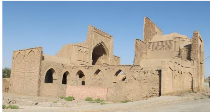
Figure 2.24. The Farumad mosque from the east
