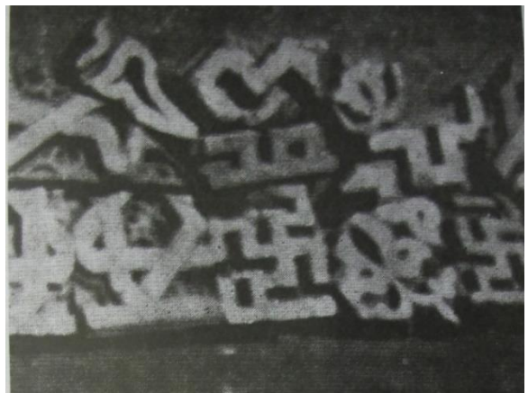
Figure 2.38. The photo of the brickwork elements of the Khosrowshir Mosque (Molavi, 1968)
