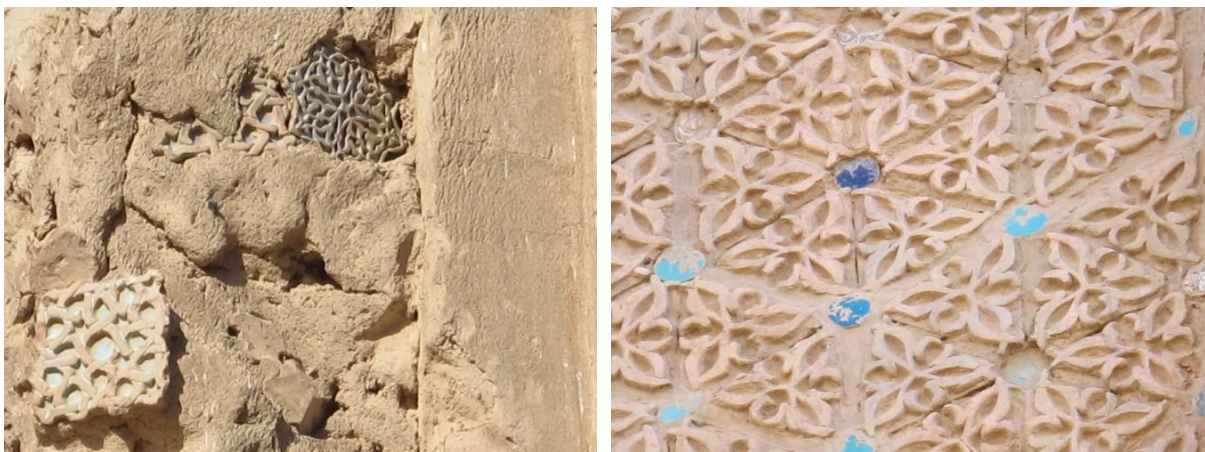
Figure 2.29. Glazed bricks at the column of the northern edge of the qibla iwan (left) and the glazed decorations at the surface of the blind arch at the right (south side) of the north-eastern iwan
