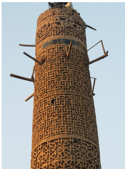
Figure 1.12. The Minaret of Masjed-e Jāme‘-e Damghān, ca. 1058 AD
