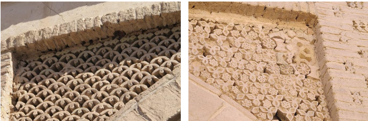
Figure 2.36. The special forms of pish-shekli elements at the spandrels of the arcades in the Masjed-e Sangān
