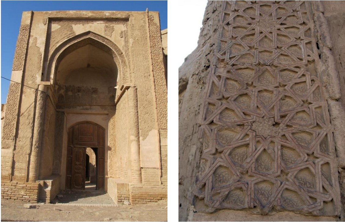
Figure 2.25. The portal of the Farumad mosque (left) and the details of its brickwork frieze
