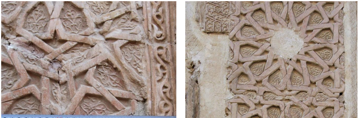
Figure 2.28. The kite-shaped bricks of the north-eastern iwan (left) and square elements of the qibla iwan (right)
