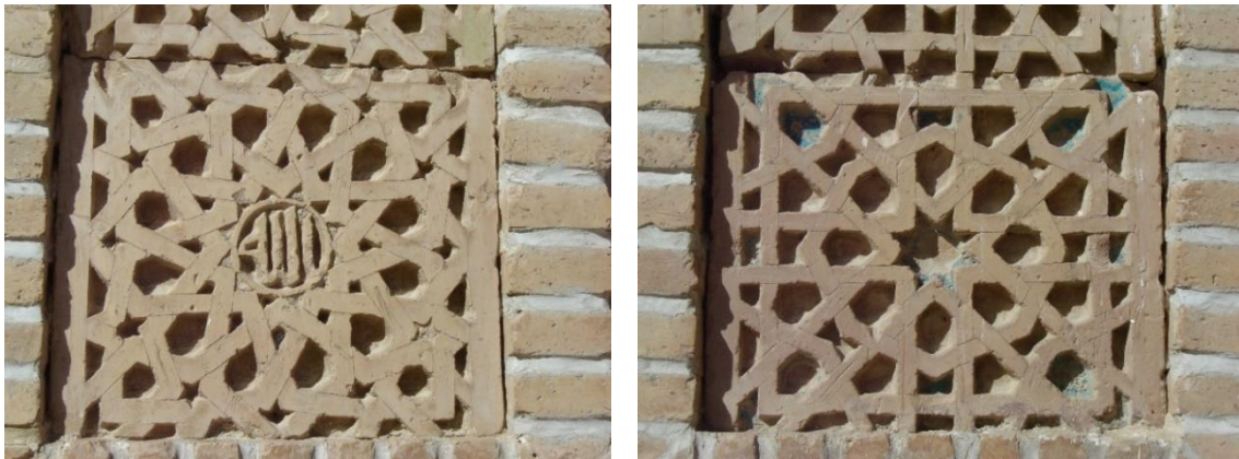
Figure 2.7. The different decorations (inscription and glazing) of the central stars on some pish-shekli bricks comparing with those adorned by glazed hobnail, (the façade of the north iwān of the Masjed-e Jame'-e Gonābād)
