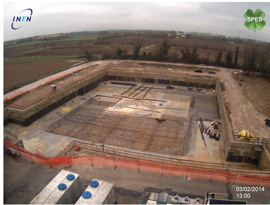
FIGURE 1.18: Photograph of excavations for the building construction at LNL.
