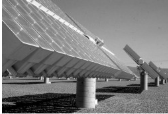
Figure 1.1 The 350-kWp SOLARAS project power plant built and deployed in Saudi Arabia by Martin Marietta using Sandia Labs technology [1].
